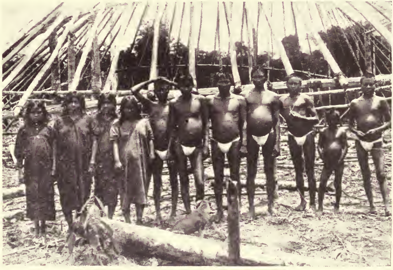
Witoto Indian group, and house in process of construction
