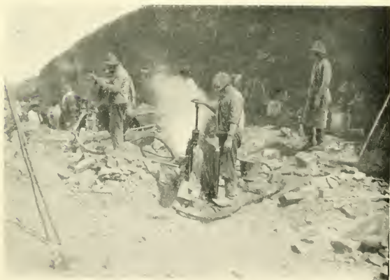
STEAM DRILL AT WORK, ARGENTINE N.E. RAILWAY EXTENSION.
