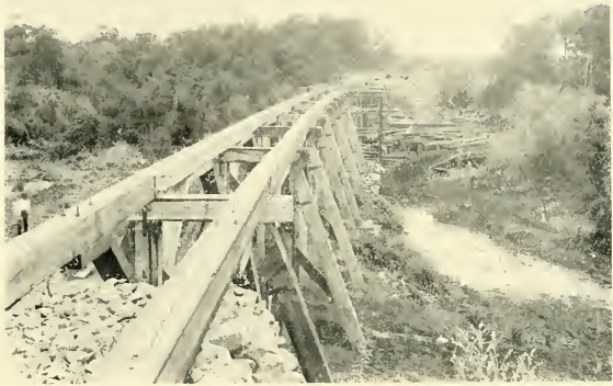
TEMPORARY BRIDGE AT BOUNDARY OF CORRIENTES AND MISIONES.
