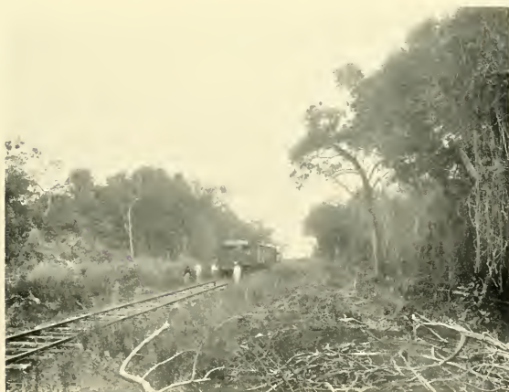
FOREST CLEARING, EXTENSION OF ARGENTINE N.E. RAILWAY TO POSADAS.
