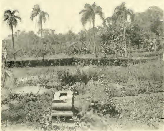
PALMS AND BROKEN MASONRY.
