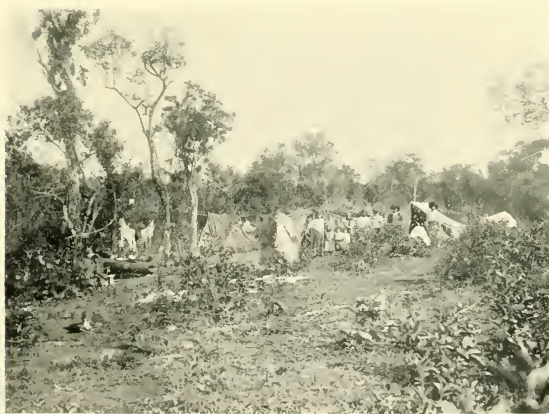
PEONES CAMP DURING RAILWAY CONSTRUCTION IN MISIONES.
