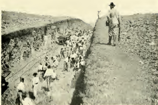
CUTTING ON ARGENTINE N.E. RAILWAY EXTENSION TO PARAGUAY.
