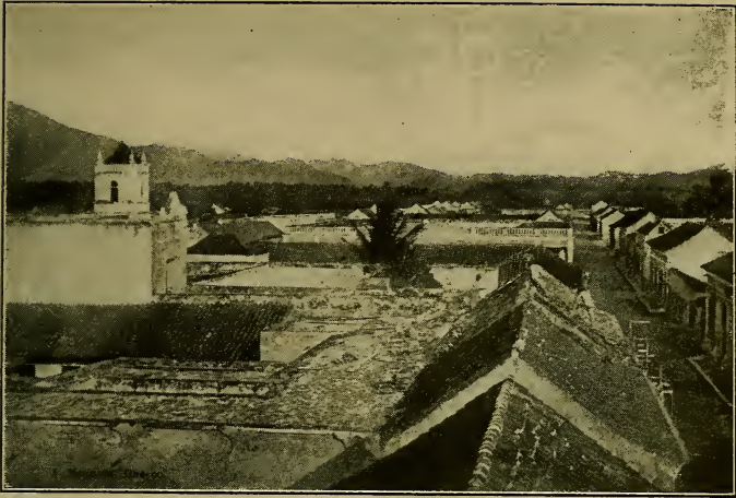
“The roofs of the houses of a whole block are joined together at all sorts of angles.”
