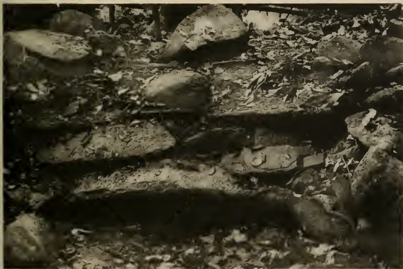
2. VIADUCT OVER SMALL STREAM, PUEBLITO
