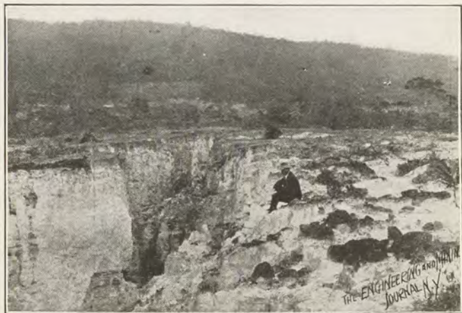
OLD WASHINGS AT MOSQUITOS, LENÇOES, Showing white shales underlying diamond bearing formations.
