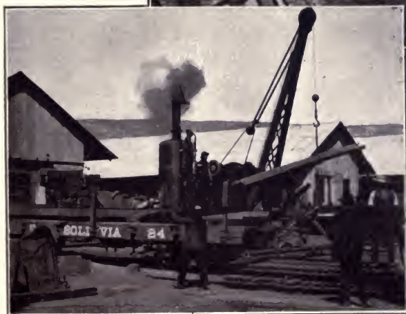
CONSTRUCTION WORK ON THE GUAQUI RAILROAD
