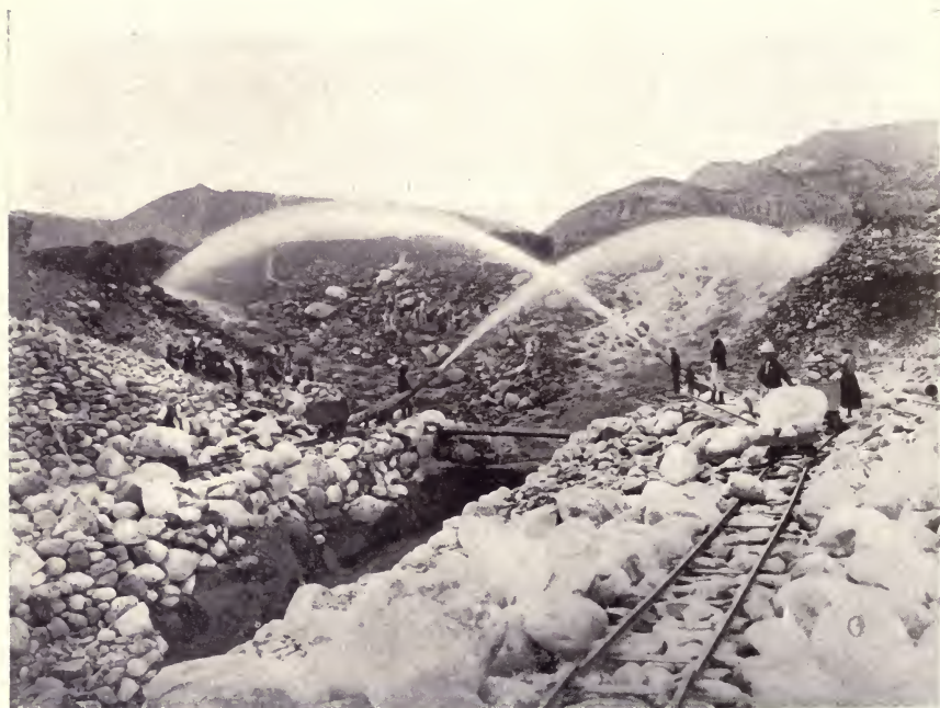
HYDRAULIC MINING IN THE CHUQUIAGUILLO RIVER
