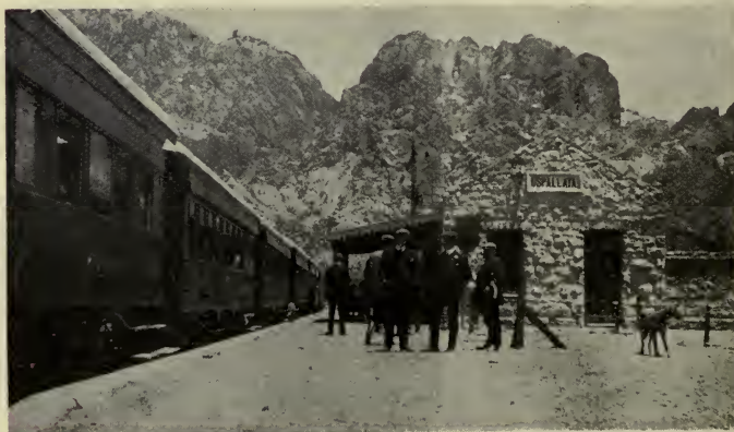
TRANSANDINE RAILWAY, USPALLATA STATION.
