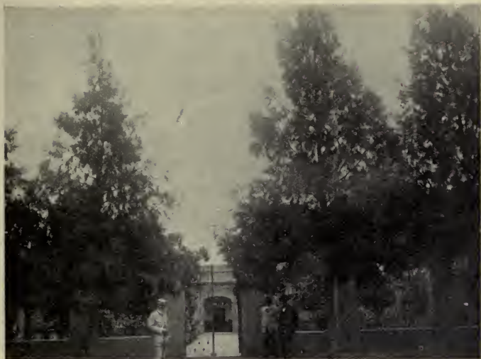
BICHADERO ESTANCIA—ENTRANCE TO COURTYARD.
