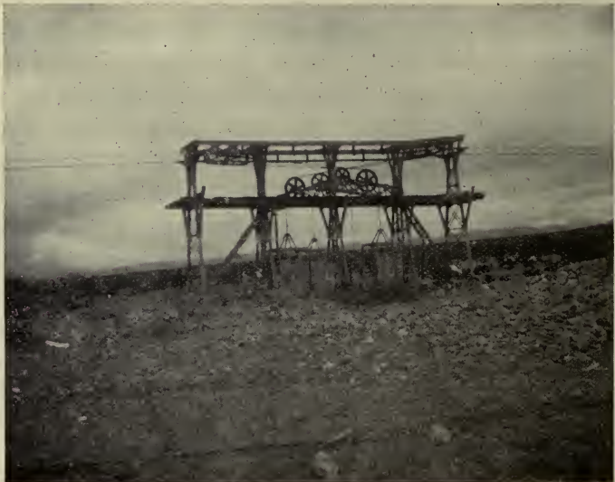
FAMATINA MINE—TENSION STATION OF AERIAL ROPE-WAY.
