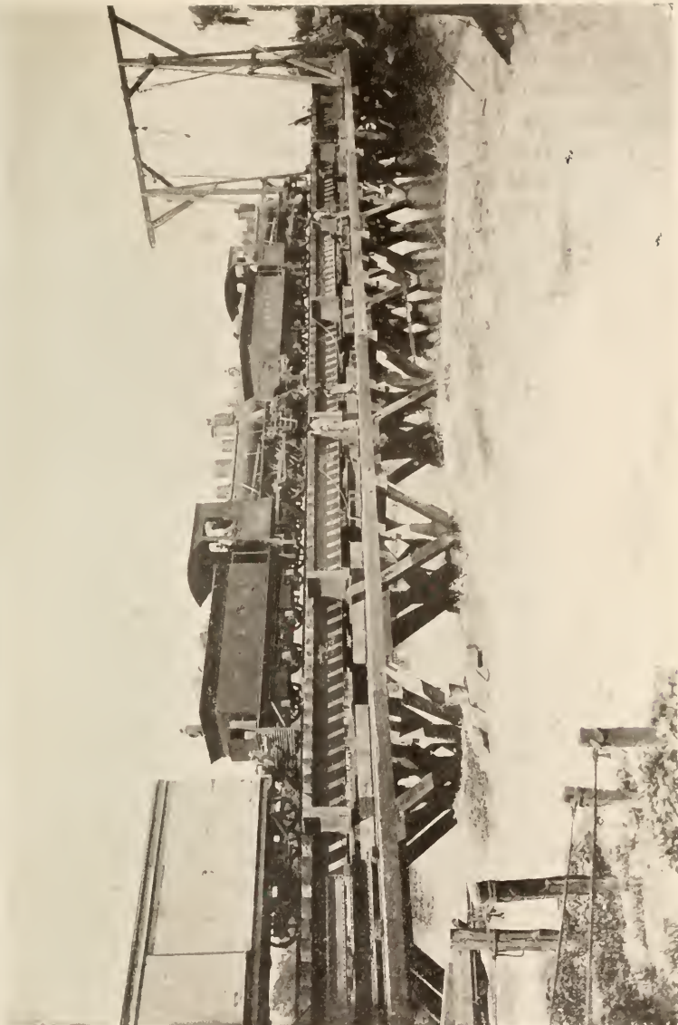
FREIGHT TRAIN FOR EXTRE RIOS CROSSING NEW BRIDGE.
