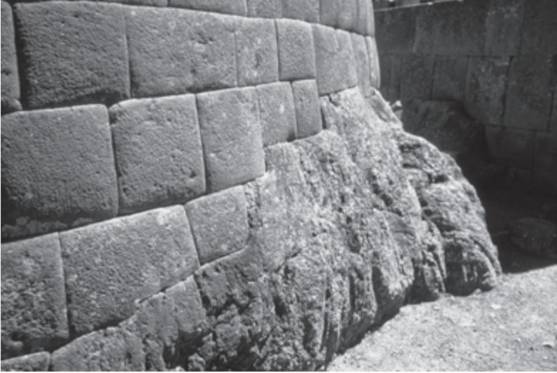
3. Outcrop integrated into a masonry wall, Písaq.
