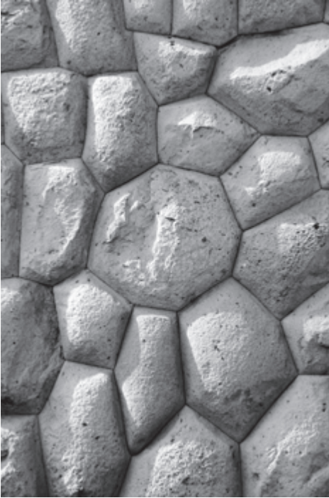
22. Uncoursed polygonal masonry, Tarawasi.
