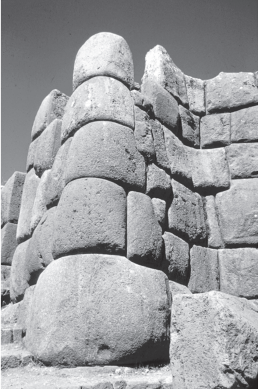
(above) 26. Polygonal and coursed masonry, Saqsaywaman.
