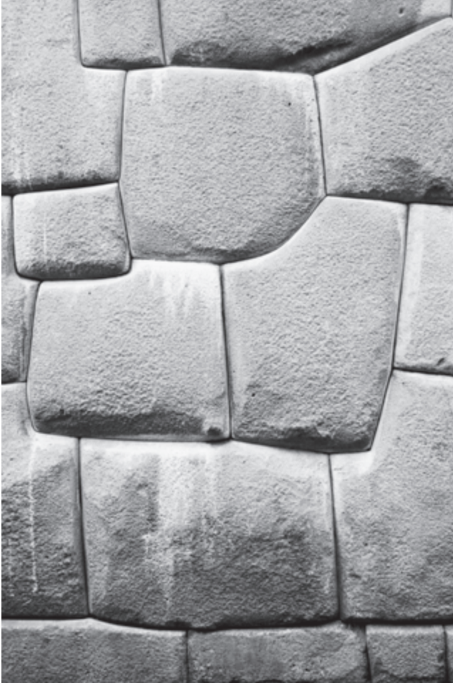
34. Pecked wall of nibbled stone, Compound of Inka Roqa (Archbishop's Palace), Cuzco.
