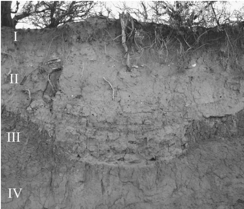
Figure 11.7 Cross section of one of the oldest irrigation canals in North America at the K'yana Chabina site (LA 48695), on the Zuni Reservation in northwestern New Mexico (from Damp et al., 2002, fig. 2; reproduced by permission of the Society for American Archaeology from American Antiquity , v. 67, no. 4, 2002; provided by J. E. Damp). The roman numerals indicate stratigraphic units described by Damp and coworkers. Unit III is a cumelic A horizon. The dark hues and fine structure show well and help to highlight the outline of the canal. The canal fill (part of Unit II) dates to ~2000yr B.P.
