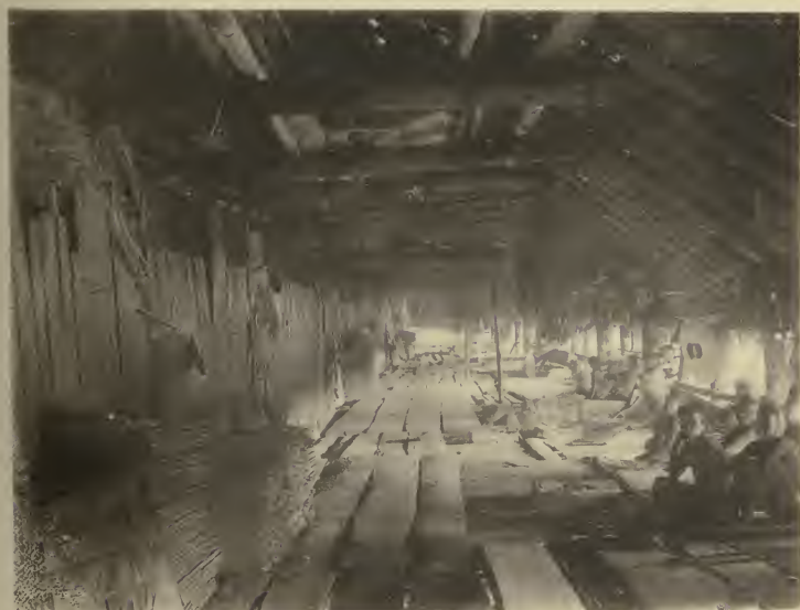
PLATE 150. GALLERY OF A KAYAN LONG HOUSE.
