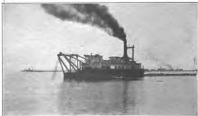
THE GREAT DREDGE, MANILA PORT WORKS.
