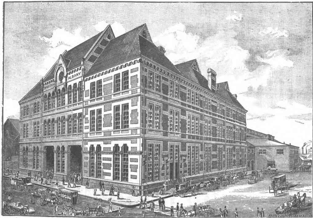
NEW DEPOT, BOSTON & ALBANY RAILROAD, KNEELAND STREET.
