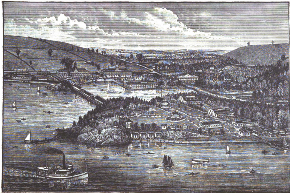
VIEW OF DOWNER LANDING.
