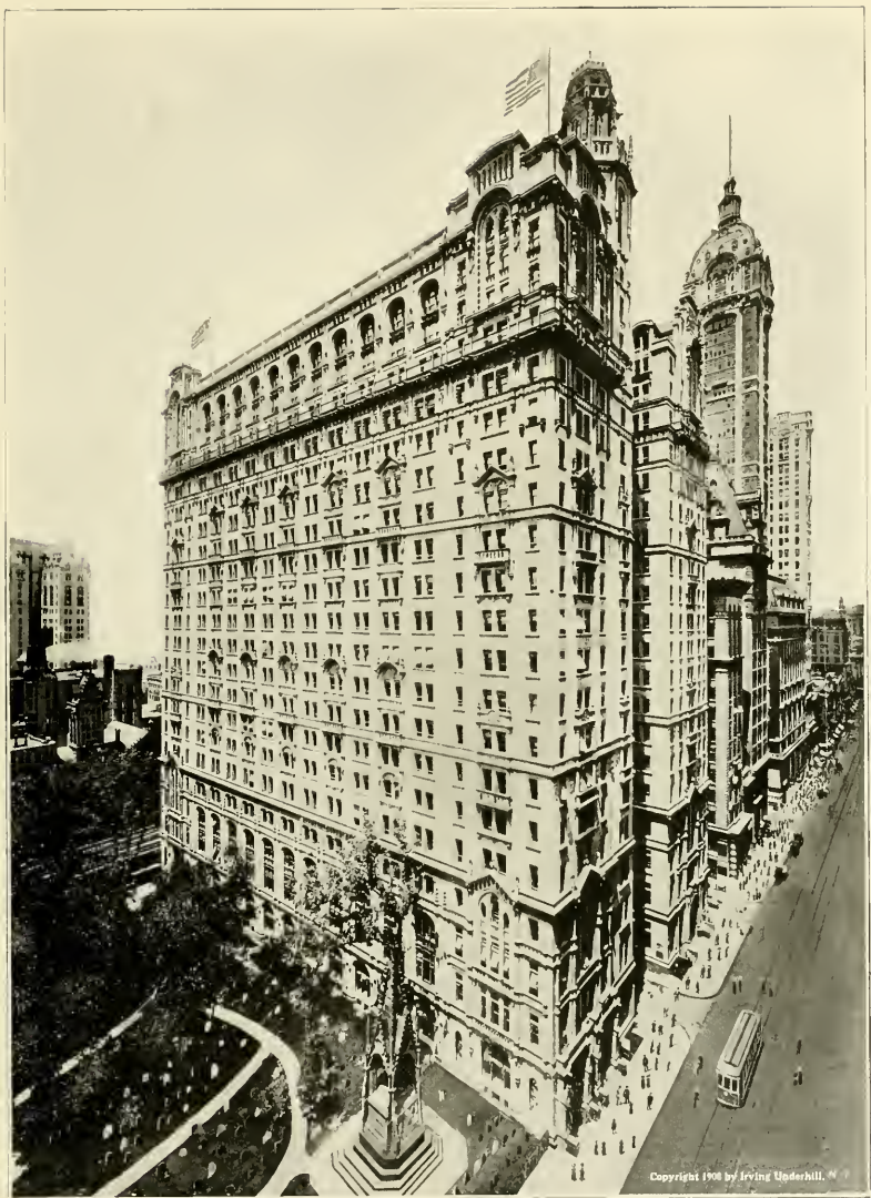
THE TRINITY BUILDING—Located at 111 Broadway just south of Trinity Church. It is a magnificent modern office building of pure Gothic architecture rising to a height of 308 feet, and resting on 70 pneumatic caissons, each one sunk 75 feet below the sidewalk.
