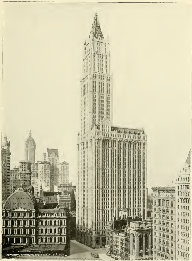
THE WOOLWORTH BUILDING—Occupies a plot 152 x 197 feet at Broadway and Barclay Street. It is the tallest building in the world rising to a height of 750 feet, 55 stories above the ground. The foundation consists of caissons 19 feet in diameter sunk to bedrock, 110 to 130 feet below the ground. Total cost is estimated at $15,000,000.
