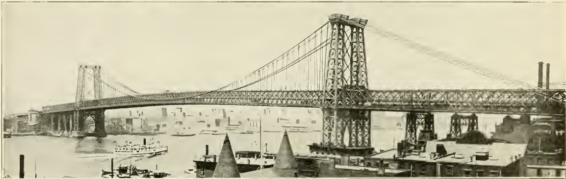
WILLIAMSBURG BRIDGE —This is a combined cantilever and suspension bridge, opened Dec. 19, 1903, crossing the East River from Delancey Street, New York City to Broadway, Brooklyn. Total length 7200 feet, width 118 feet, height 135 feet above the water. Cost $10,000,000.
