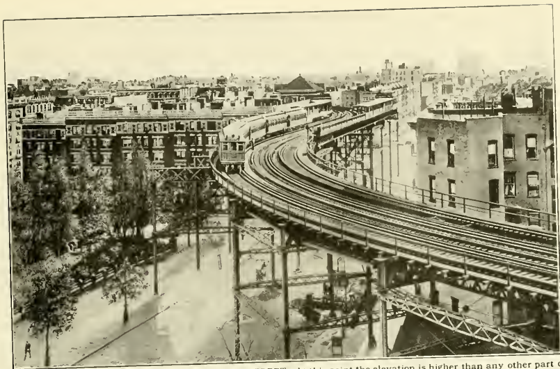
ELEVATED RAILWAY CURVE AT 110TH STREET —At this point the elevation is higher than any other part of the city, reaching a height equal to five stories and requiring elevators at the station to take up and down the passengers. New York City is famous for its elevated Railroads, this being one of the most noted sections.
