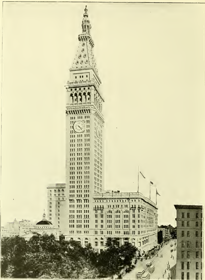
METROPOLITAN LIFE INSURANCE BUILDING —Located at No. 1 Madison Avenue, opposite Madison Square. It is built of carved white marble and is the most elegantly finished and valuable building in the world. The tower is 700 feet high, 52 stories. The electric clock is 30 feet in diameter and at night is visible for miles.
