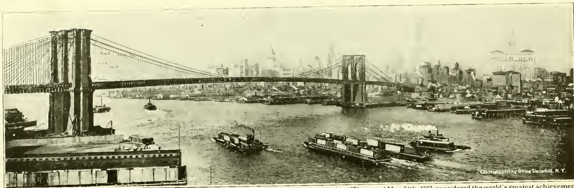
BROOKLYN BRIDGE —From City Hall, Manhattan, to Sands St., Brooklyn. Bridge was started in 1870, opened May 24th, 1883, considered the world's greatest achievement in bridge construction. Total length, 6537 feet, width 85 feet. 500,000 people and 5,000 vehicles cross the bridge daily.
