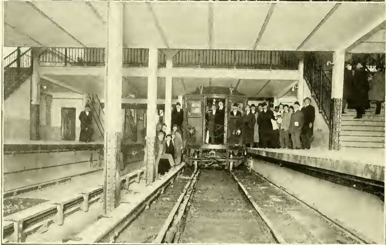
BROOKLYN BRIDGE SUBWAY STATION —New York City's Subway System is the most complete of any in the world. The Brooklyn Bridge Station is the busiest in the world. It is estimated that 2,000,000 pass here daily. The subway contains 4 tracks, 2 for express trains and 2 for local trains. During the rush hours the trains are run on a one minute schedule.
