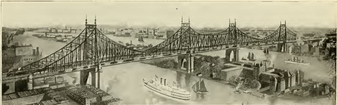
BLACKWELL'S ISLAND BRIDGE —Over the East River from East 59th Street and 2nd Avenue, Manhattan, to Jane and Academy Streets, Long Island City. A great cantilever structure costing, with approaches, $25,000,000; 7,636 feet long, west span, 1,182 feet; clear height over channels, 135 feet; width 86 feet, two decks with 53 foot road.
