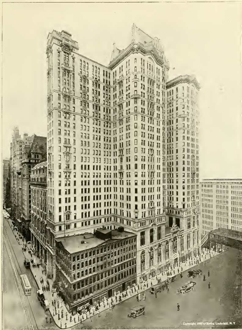
THE CITY INVESTMENT BUILDING —This mammoth structure, located on Broadway between Cortlandt and Church Streets, is the most spacious office building in the world. It covers a plot of 27,000 square feet, contains 13 acres of floor space and has room for 6,000 tenants. It rises 34 stories above the sidewalk, a total height of 486 feet. Total cost $10,000,000.
