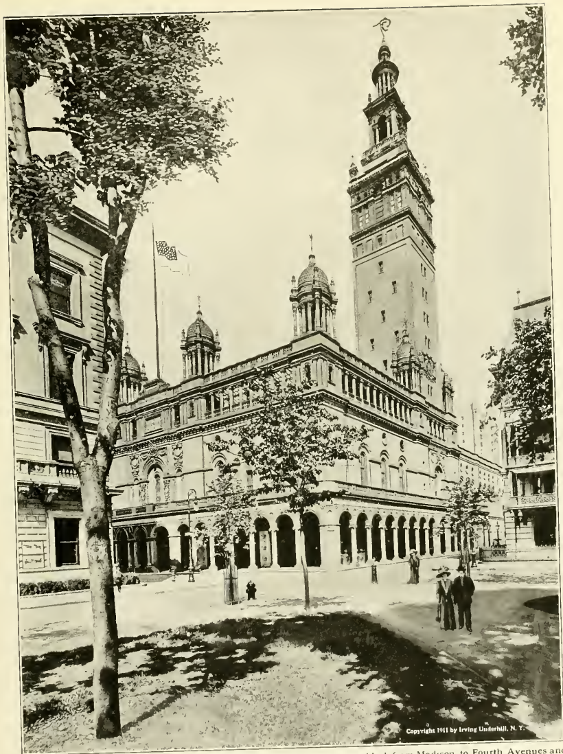
MADISON SQUARE GARDEN —This building occupies an entire city block from Madison to Fourth Avenues and 36th to 37th Streets. It is the largest Amphitheatre in America, the interior being 300 by 200 feet, 80 feet high, with an arena 268x122 feet, seating capacity 12,000. The tower is 341 feet high, statue of Diana is 13 feet high. Erected in 1890 at a cost of $3,000,000.
