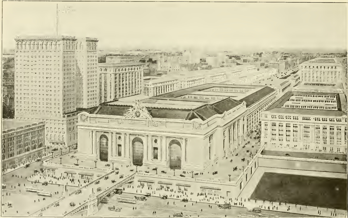
THE GRAND CENTRAL TERMINAL—Covers 69.8 acres facing East 42nd St., from Vanderbilt to Lexington Ave., the largest and most costly Railroad Station in the world. It has 31 miles of tracks under cover, with a capacity for handling 200 trains and 70,000 passengers each hour. There are 42 tracks for long distance express trains on the 42nd Street level, and 25 tracks for suburban trains in concourse, 25 feet below the street.
