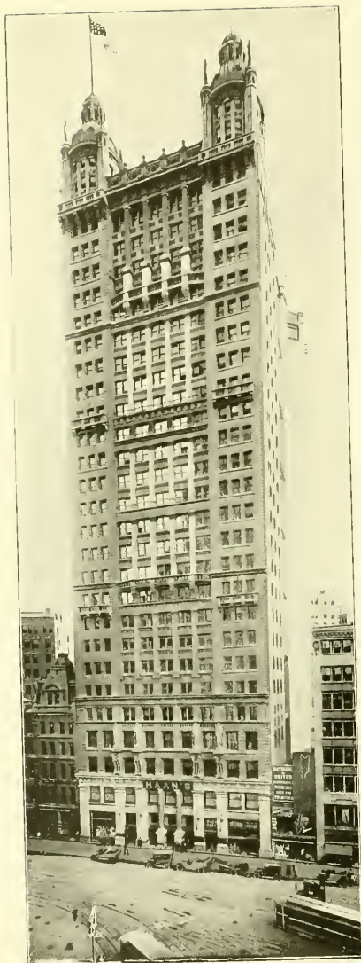
PARK ROW BUILDING —Located at the head of Park Row, opposite the General Post Office adjoining Ann St. It rises to a height of 29 stories including tower, 381 feet high. It is built entirely of lime stone and has the distinction of being the first skyscraper in New York, being ready for occupancy in October, 1899. Total cost, $3,500,000.
