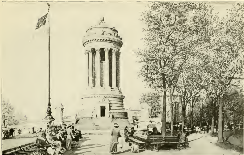
THE SOLDIERS AND SAILORS MONUMENT —Is situated on Riverside Drive near 89th Street. It is built of beautiful white marble, about 90 feet high. The columns in the center, of which there are 10, being 35 feet high.
