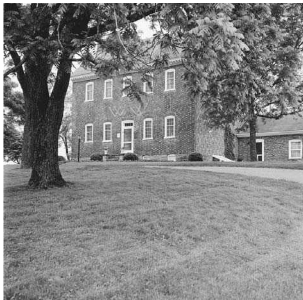
William Whitley House. Built between 1787 and 1794, the William Whitley house in Stanford, Kentucky, is believed to be the oldest brick residence west of the Allegheny Mountains.
