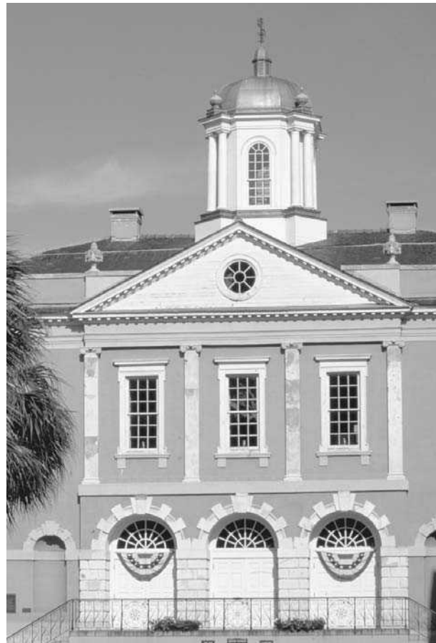
The Exchange and Provost Dungeon. Charleston’s Exchange was built in 1767 to 1771 after the adoption of the Townshend Acts, which mandated duties on imports of glass, lead, painters’ colors, tea, and paper. The Exchange had commodious cellars for customs storage; during the British occupation, American prisoners were held there. © JAN BUTCHOFSKY-HOUSER/CORBIS.
