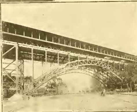
Subway Extension at 129th Street.
