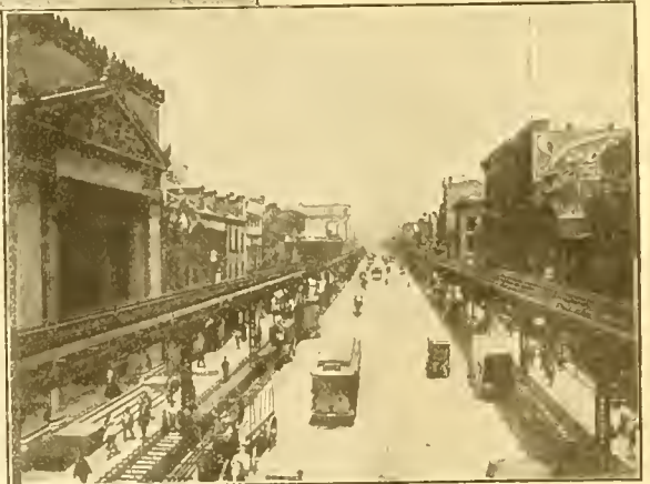
The Elevated Road on the Bowery.
