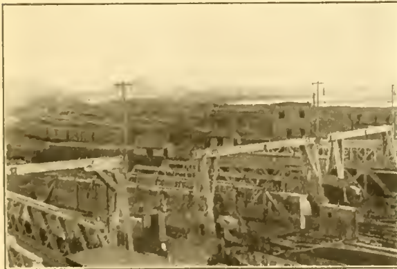
Freight Depot, New York & New Haven Railroad, The Bronx.
