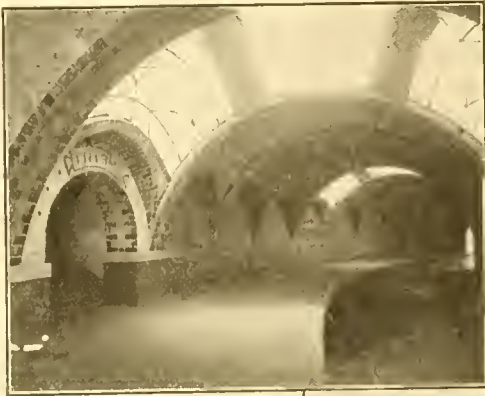
Subway at City Hall Entrance.
