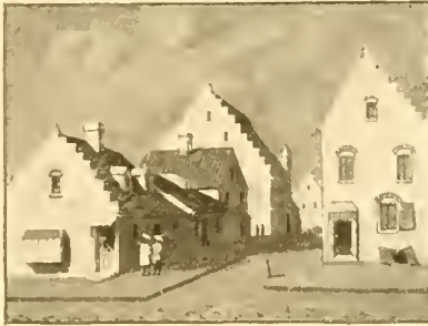
Old Dutch houses, with notches on the gable ends by which the chimney sweeps could climb.
