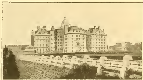
St. Luke's Hospital.
