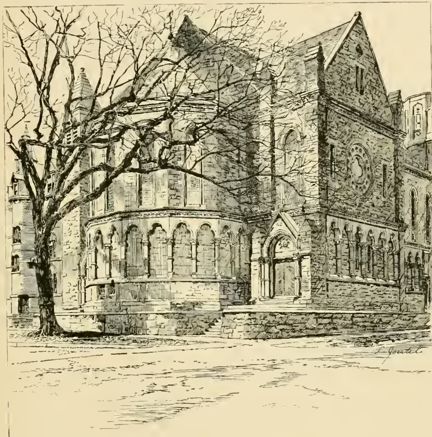
REAR OF THE CHAPEL
