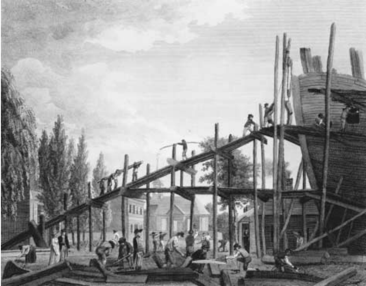
Construction of the Philadelphia . During the era of the Napoleonic Wars, war with either France or England appeared imminent, and a number of frigates were built in response, including the Philadelphia , shown under construction in Philadelphia in the late 1790s in this engraving by William and Thomas Birch. I. N. PHELPS STOKES COLLECTION, MIRIAM AND IRA D. WALLACH DIVISION OF ART, PRINTS, AND PHOTOGRAPHS, NEW YORK PUBLIC LIBRARY, ASTOR, LENOX AND TILDEN FOUNDATIONS.
