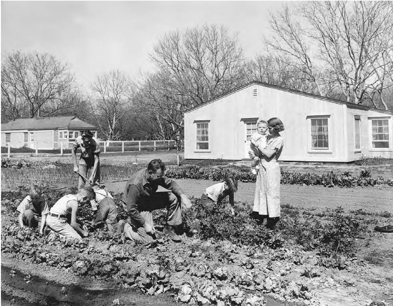
Members of a family of eight work in their garden at the El Monte federal subsistence homesteads in California in 1936. The father, a streetcar conductor whose monthly pay was one hundred dollars, paid sixteen dollars and twenty cents per month toward purchase of the four-bedroom house seen in the background. LIBRARY OF CONGRESS, PRINTS & PHOTOGRAPHS DIVISION, FSA/OWI
