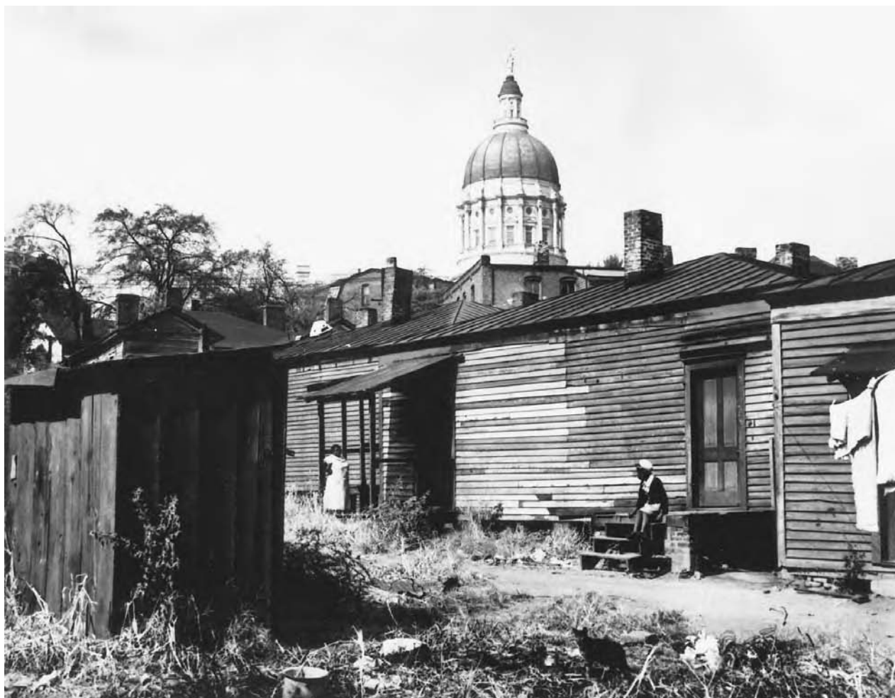
These dilapidated buildings stood on the Georgia State Capitol Homes site in Atlanta, Georgia, before the U.S. Housing Authority demolished them and began a construction project on the site during the late 1930s. FRANKLIN DELANO ROOSEVELT LIBRARY
