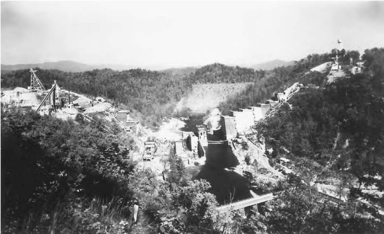
The Hiawasse Dam in North Carolina, under construction by the TVA in the late 1930s. FRANKLIN DELANO ROOSEVELT LIBRARY
