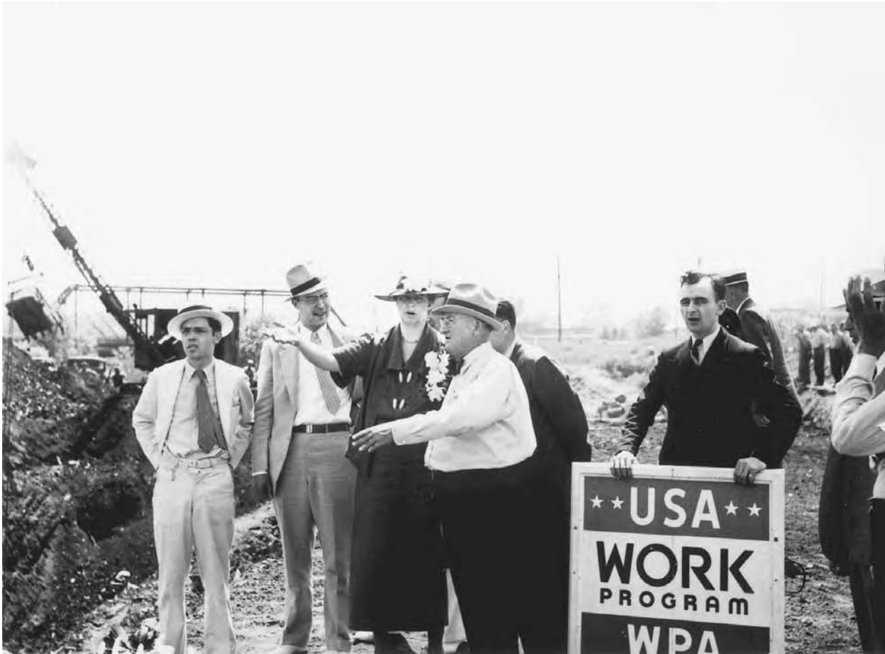
Eleanor Roosevelt visits a WPA construction site in Des Moines, Iowa, in June 1936. FRANKLIN DELANO ROOSEVELT LIBRARY
