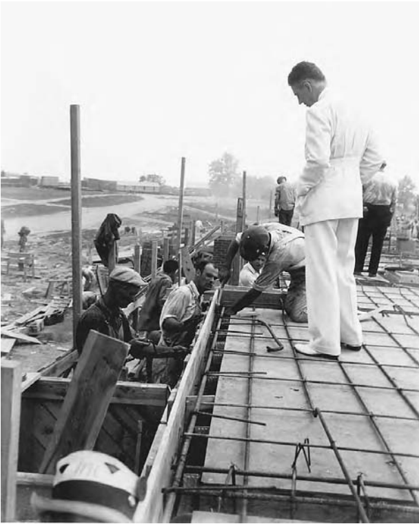
Rexford Tugwell (standing) inspects the foundations of houses under construction at the Greenbelt project in Maryland in 1936. LIBRARY OF CONGRESS, PRINTS & PHOTOGRAPHS DIVISION, FSA/OWI COLLECTION
