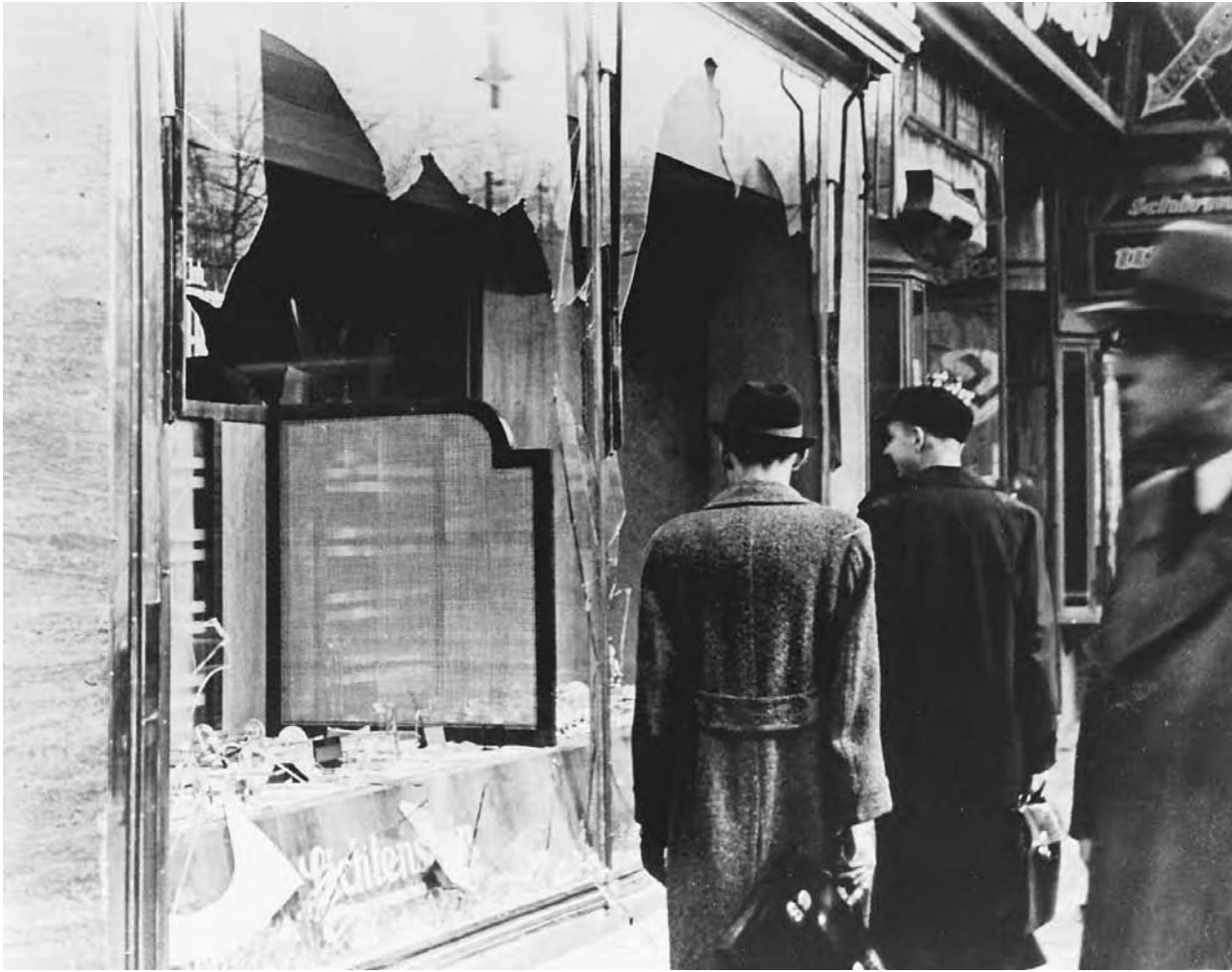
Pedestrians in Berlin pass by the shattered window of a Jewish-owned shop that was destroyed in November 1938 during Kristallnacht. NATIONAL ARCHIVES AND RECORDS ADMINISTRATION, COURTESY OF UNITED STATES HOLOCAUST MEMORIAL MUSEUM PHOTO ARCHIVES
