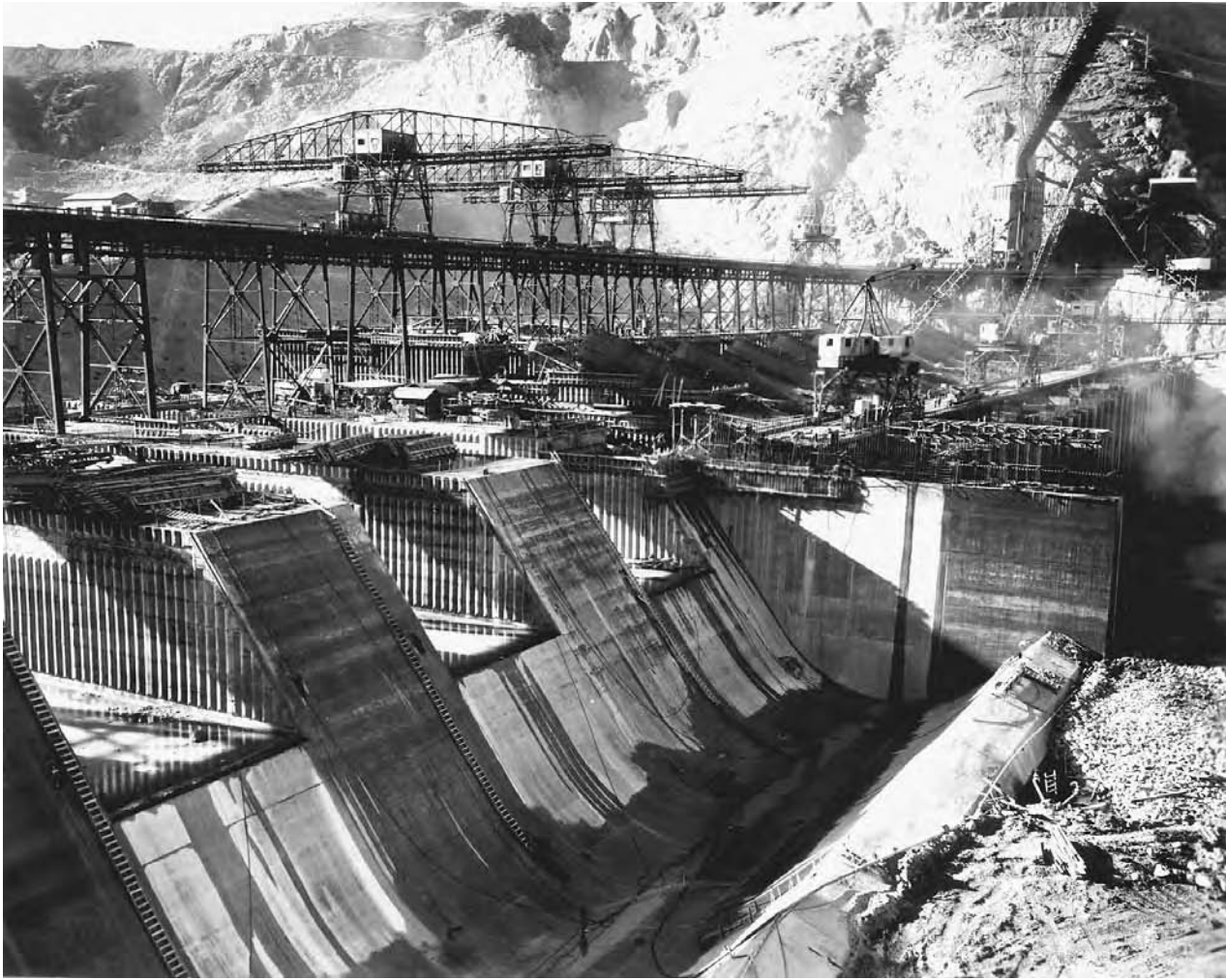
The massive Grand Coulee Dam, under construction in 1936 on the Columbia River in Washington. LIBRARY OF CONGRESS, PRINTS & PHOTOGRAPHS DIVISION, FSA/OWI COLLECTION
