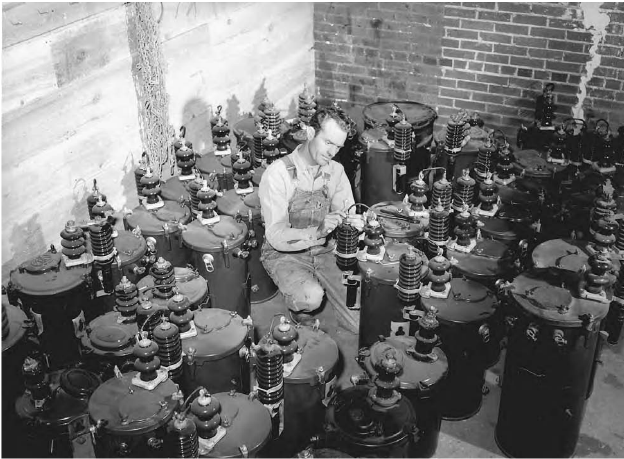
An REA employee checks transformers at the REA cooperative headquarters in Hayti, Missouri, in 1942. LIBRARY OF CONGRESS, PRINTS & PHOTOGRAPHS DIVISION, FSA/OWI COLLECTION
