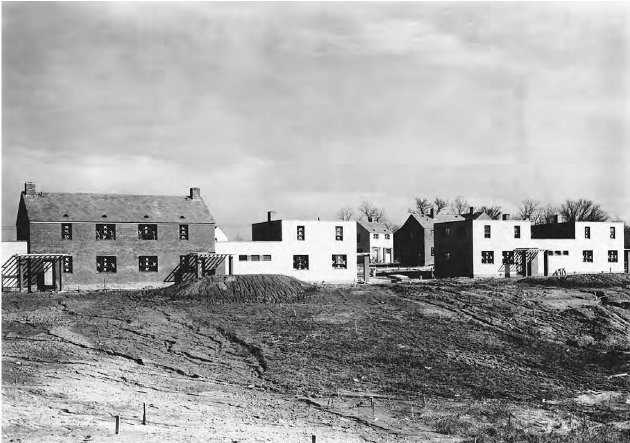
This housing project under construction in Greenhills, Ohio, in 1937 was one of numerous Resettlement Administration initiatives.
