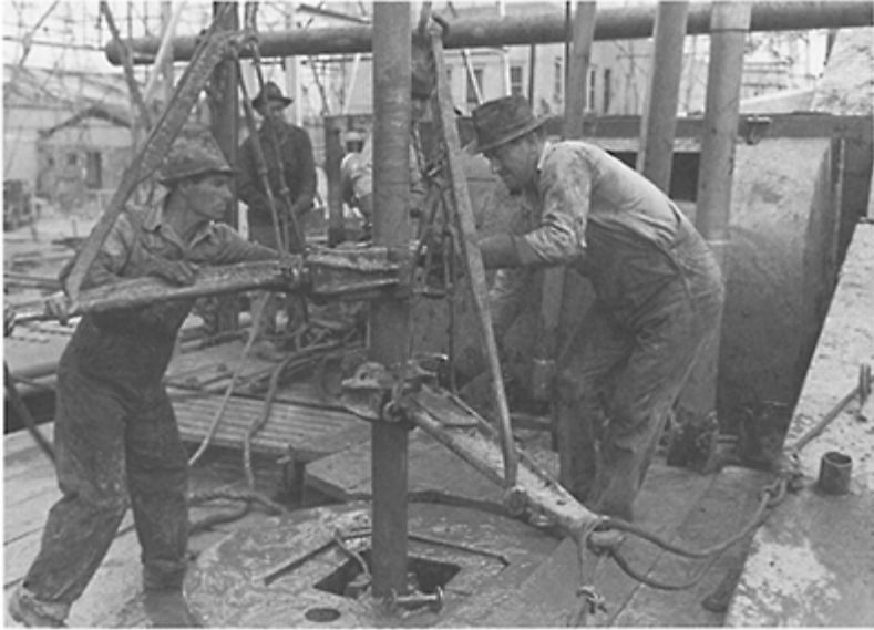
To drilla tuell, roughnecks use pipe wrenches to screw one piece of drillpipe into another. Kilgore, Texas, 1939. Photo Russell Lee. Library of Congress.
