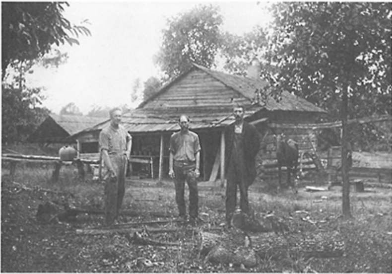
The pottery shop of Robert Ritchie (r.), Catawba County, North Carolina, ca. 1914. To the left rear is the groundhog kiln, at the back center is the log shop, and to the right is the pug mill for grinding the clay. Photo courtesy Clara Ritchie Wiggs.
