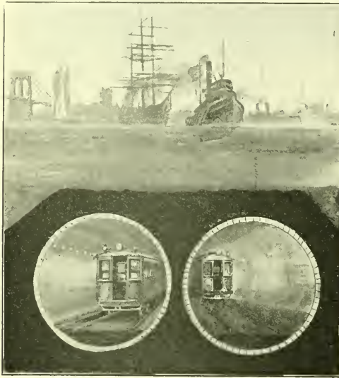
EAST RIVER SUBWAY TUNNEL
