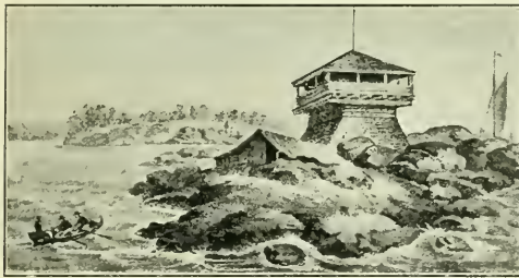
MILL ROCK, HELL GATE (1814)
