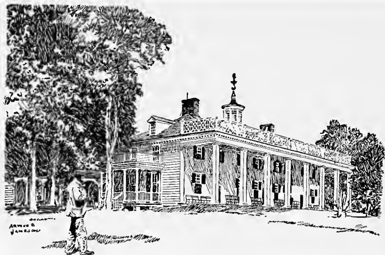
WASHINGTON'S MANSION—SOUTH AND WEST FRONTS—MT. VERNON, VA.
