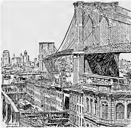
BROOKLYN BRIDGE. ONE OF THE LARGEST SUSPENSION BRIDGES IN THE WORLD.
