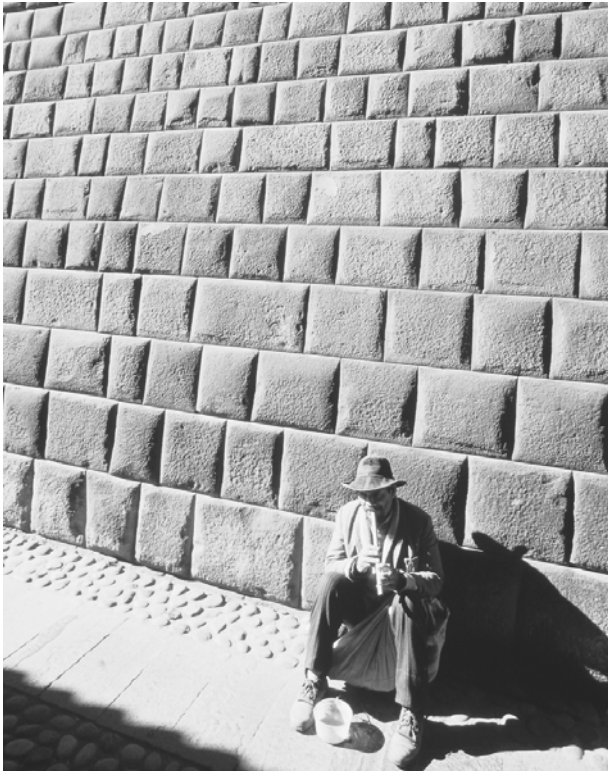
This Inca stone wall, still standing in Cuzco, shows the precision with which the Incas cut and fit each stone. © Nevada Wier/Corbis.
