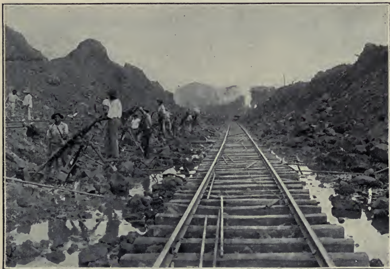
“MEN AT WORK DRILLING HOLES FOR THE CHARGES.”
