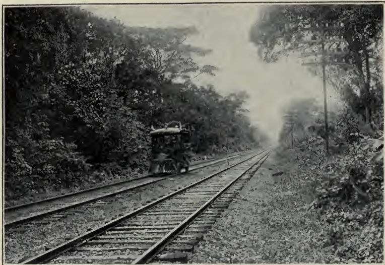
“NOW THE ROAD IS IN FIRST-CLASS CONDITION.” Private car of Chairman of Isthmian Canal Commission.
