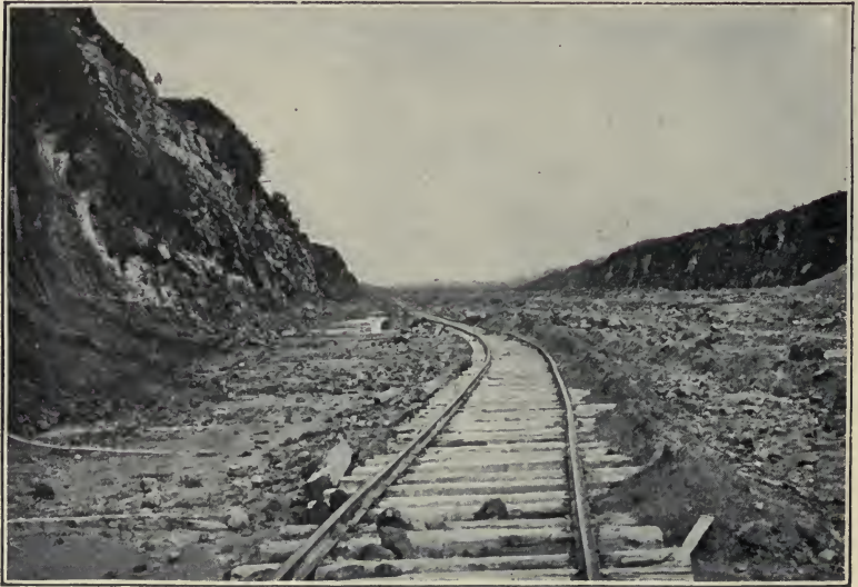
EXCAVATION FOR GATUN LOCKS COMPLETED.
