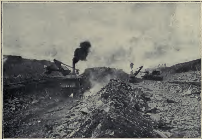
EXCAVATING FOR GATUN LOCKS.
