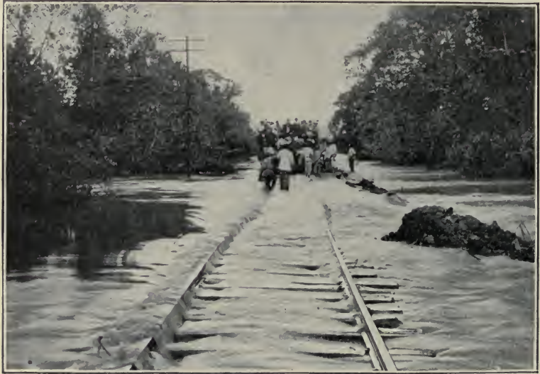
FLOODS ON PANAMA RAILROAD—1906.
