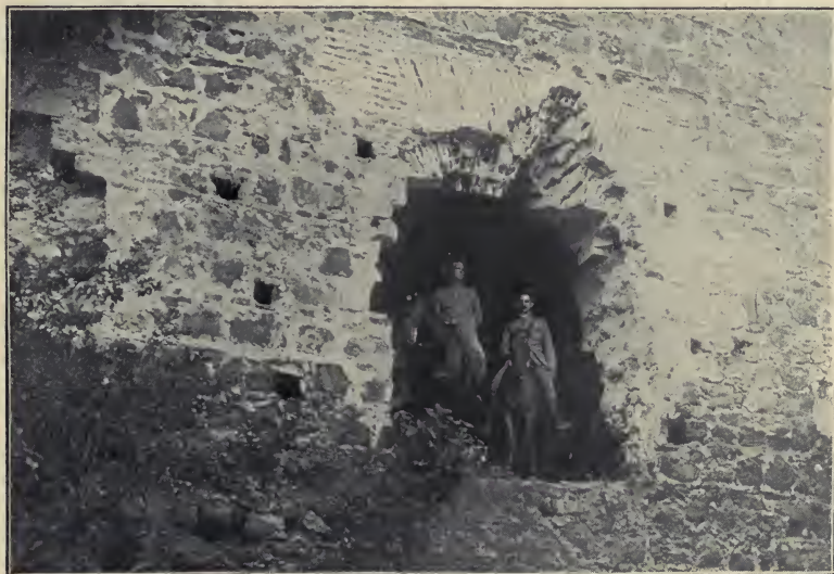
WALL OF TOWER OF ST. AUGUSTIN.—NOTE THICKNESS OF MASONRY.
