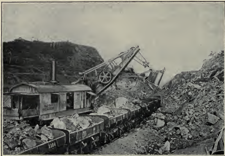
LOADING DIRT TRAIN BY STEAM SHOVEL.
