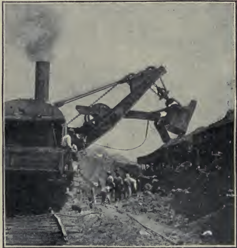
STEAM SHOVEL—SHOWING ARM AND DIPPER.
