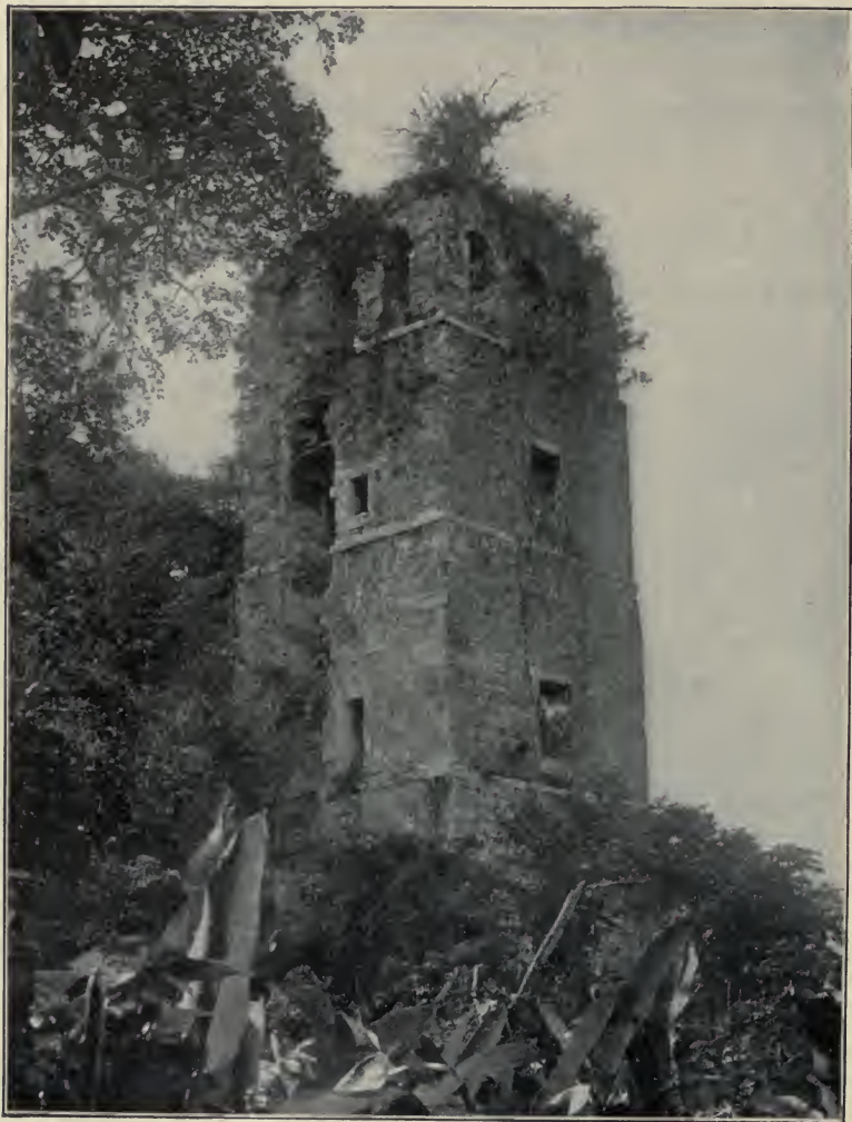
MASSIVE TOWER OF SAINT AUGUSTIN.
