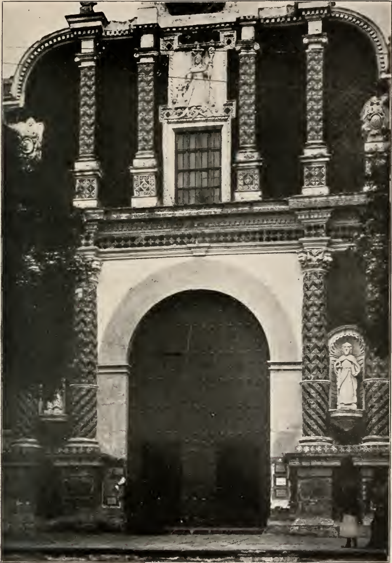
51. FRONT OF CHURCH OF SAN JOSÉ, PUEBLA. Showing Tile Pillars. Decorated in Polychrome.
