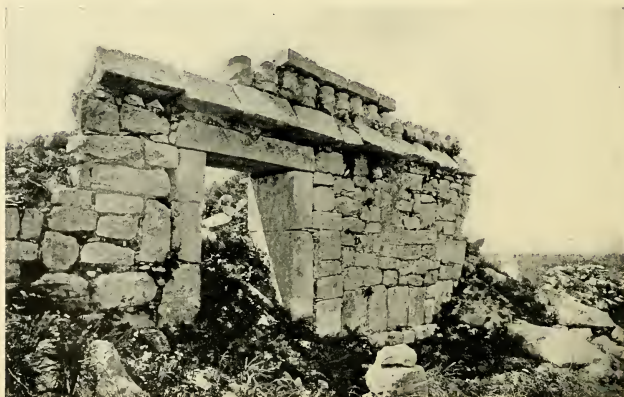
All that remains of the third story of the Nunnery. Several inscribed stones built hit or miss into the wall were doubtless taken from the older city.
