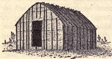
FIG. 2.—Bark house. Method of construction of the Iroquois long house. (From Handbook of American Indians.)
