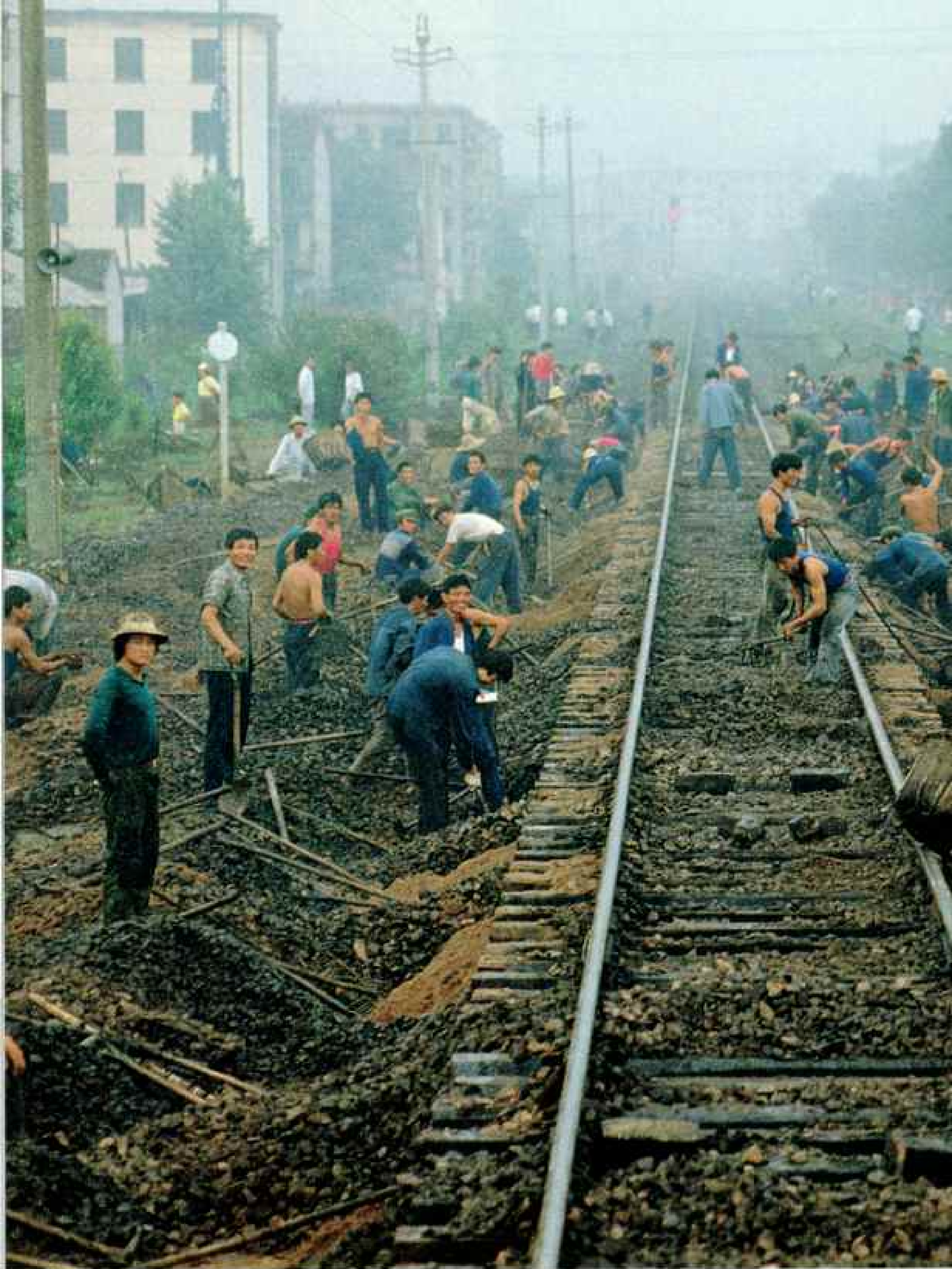
Pool of laborers, parted by the passage of the Changsha-Shanghai train, resumes work in its wake. They restore rock ballast to the railbed in
