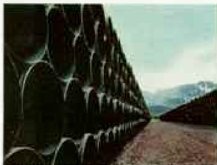
It took over one-half million tons of steel to make the 798 miles of pipe for the project. The sections are 40' and 60' long, 48" in diameter.
