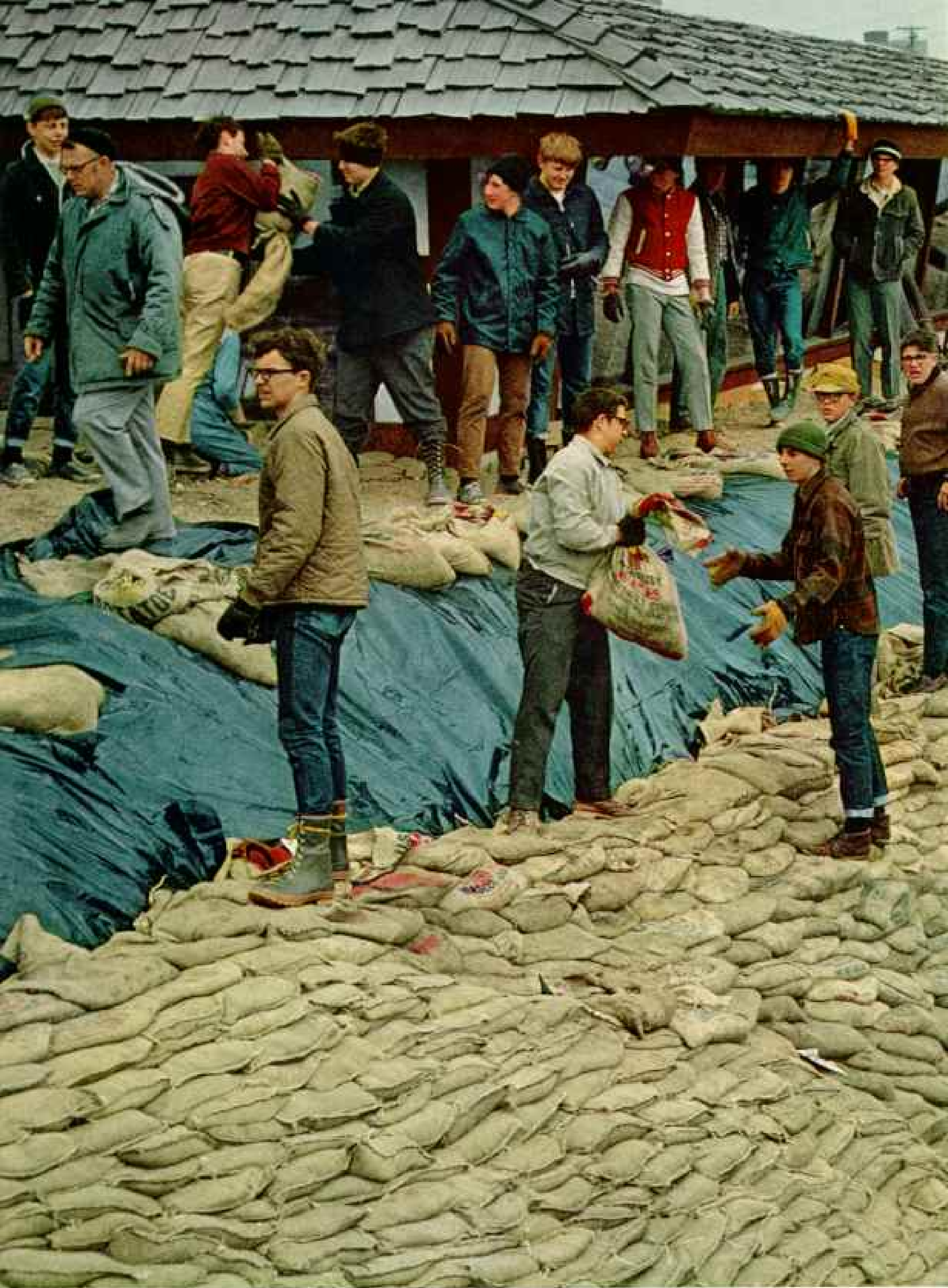
Forewarned, forearmed: A battlement climbs toward the eaves of the Century Club Restaurant in North Mankato to stave off the rising Minnesota River. Sandbags anchor sheets of polyethylene plastic to prevent scouring by currents. Most of the workers are teen-agers—
