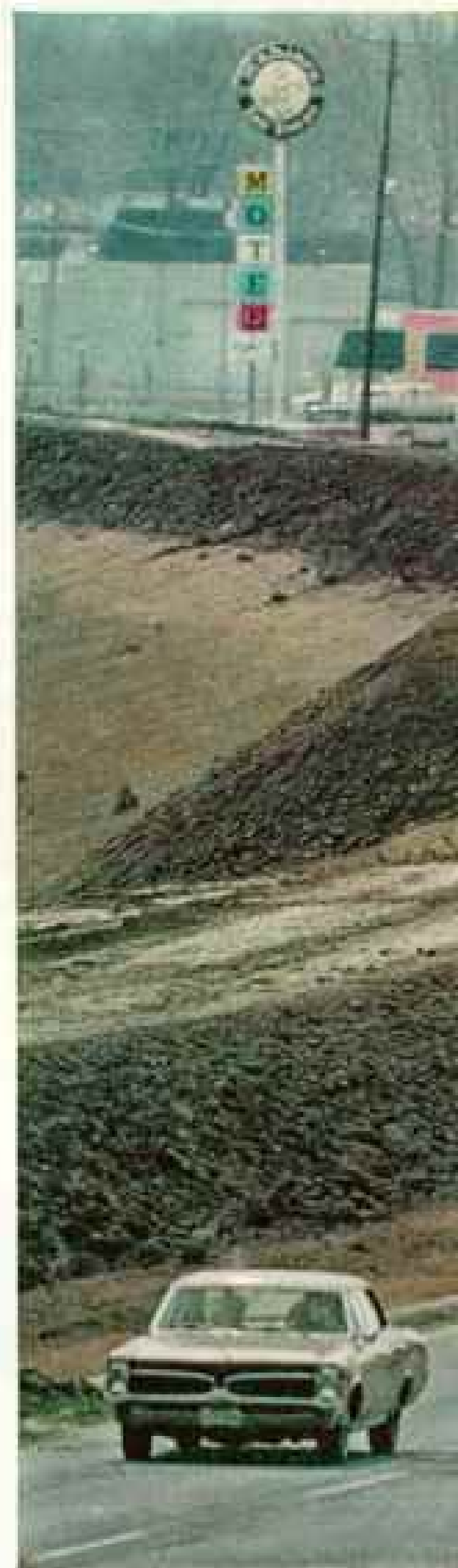
Ramparts rise atop a highway to protect North Mankato; trucks shuttle more clay
