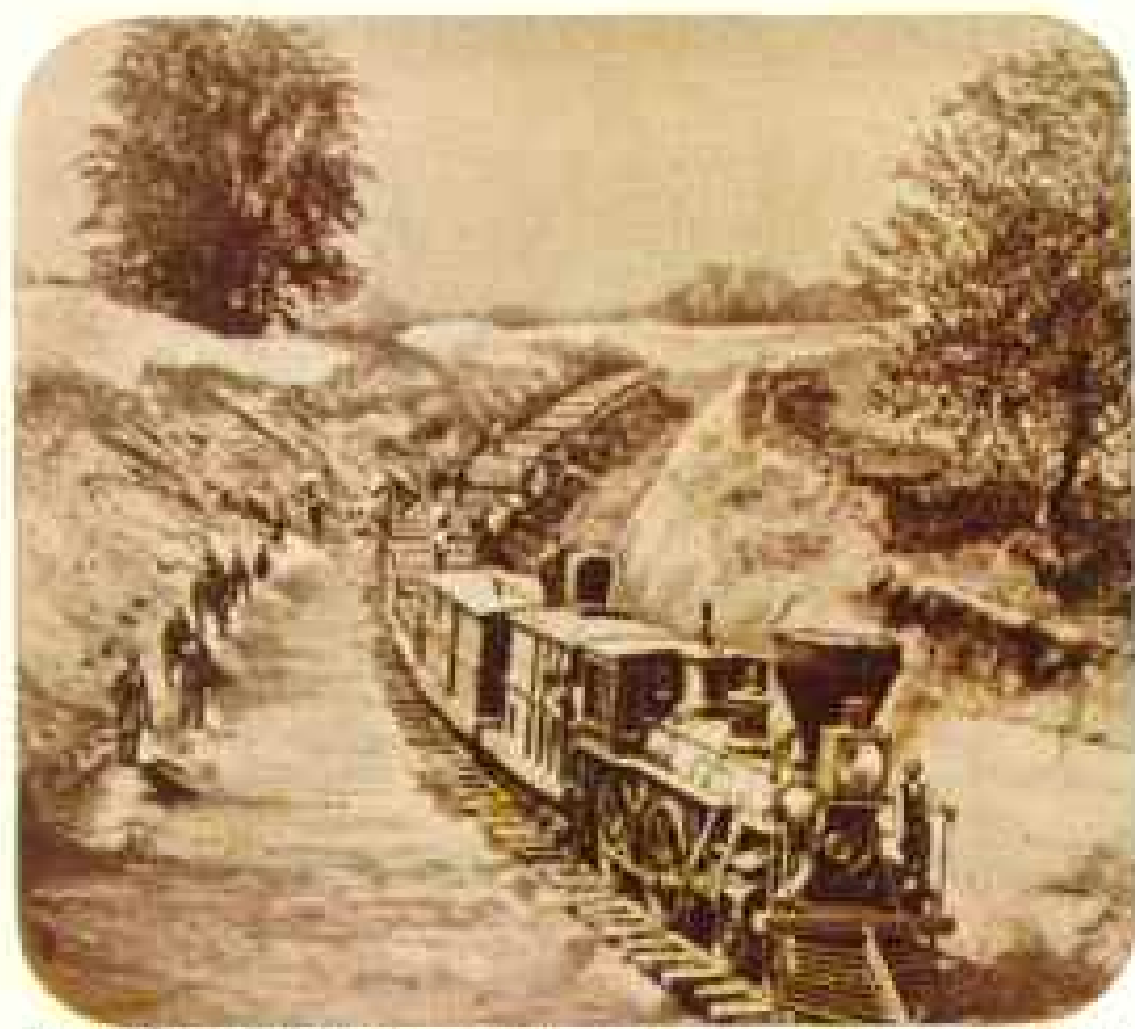
NO HUGE STEAM SHOVELS to help early Pennsylvania Railroad builders! It was pick, shovel and muscle—as you can see from this old photograph.
