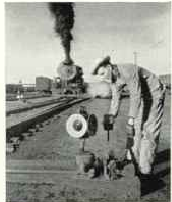
A switchman throws a switch for an oncoming yard engine with cars for assembly into a train.
