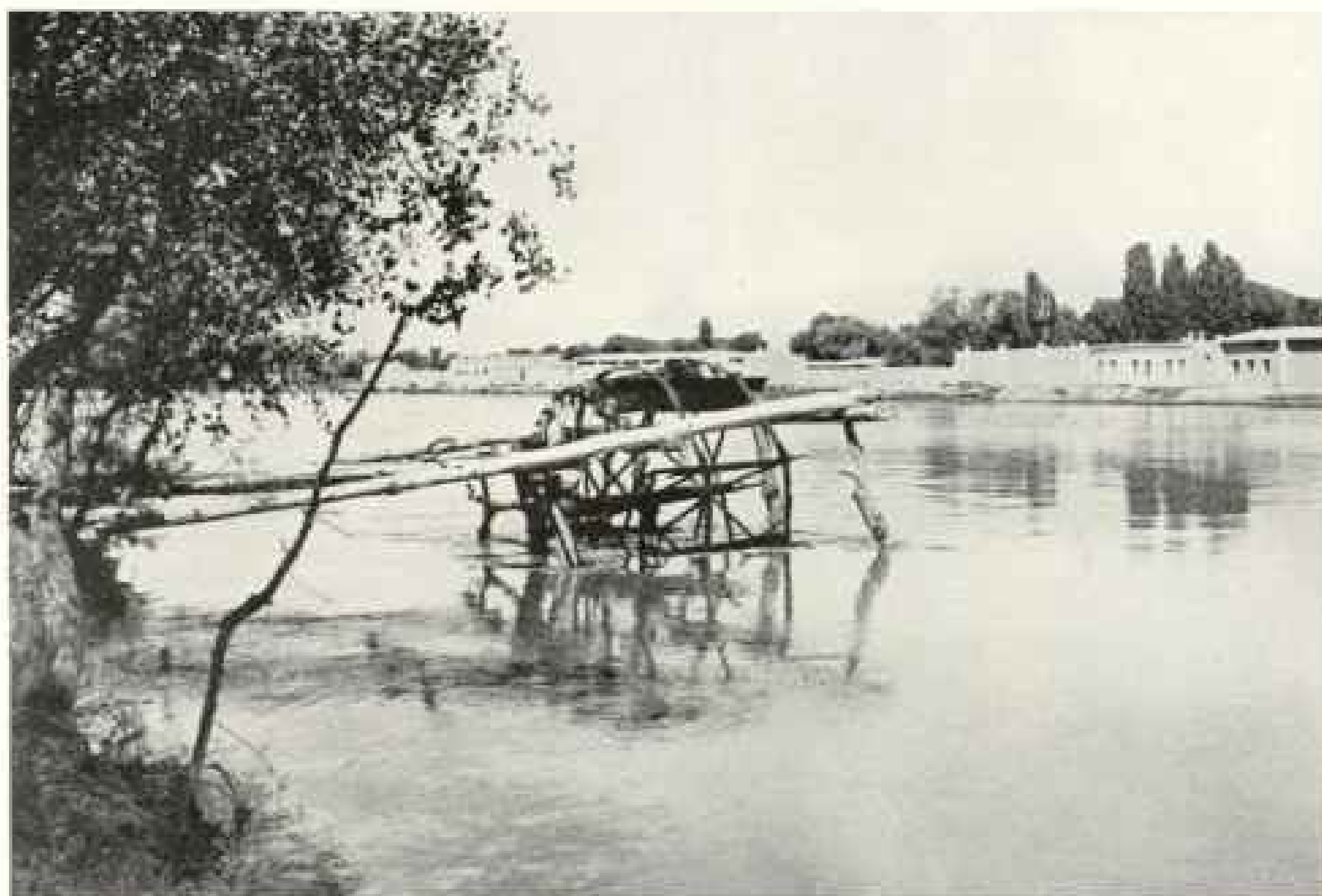
A PRIMITIVE WATER WHEEL FURNISHES POWER FOR A GRISTMILL.
