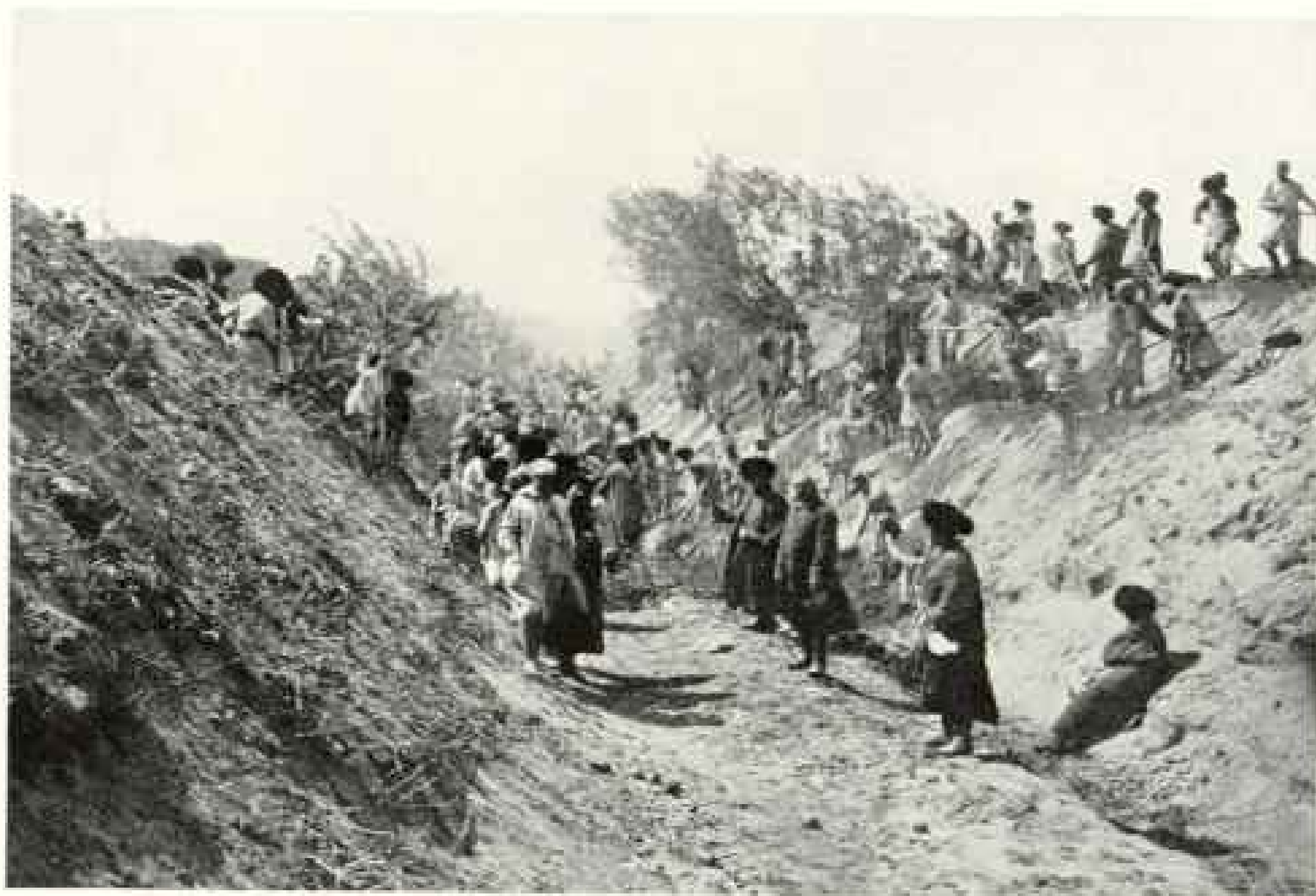
REMOVING SILT FROM A CANAL, IN KHORESM
