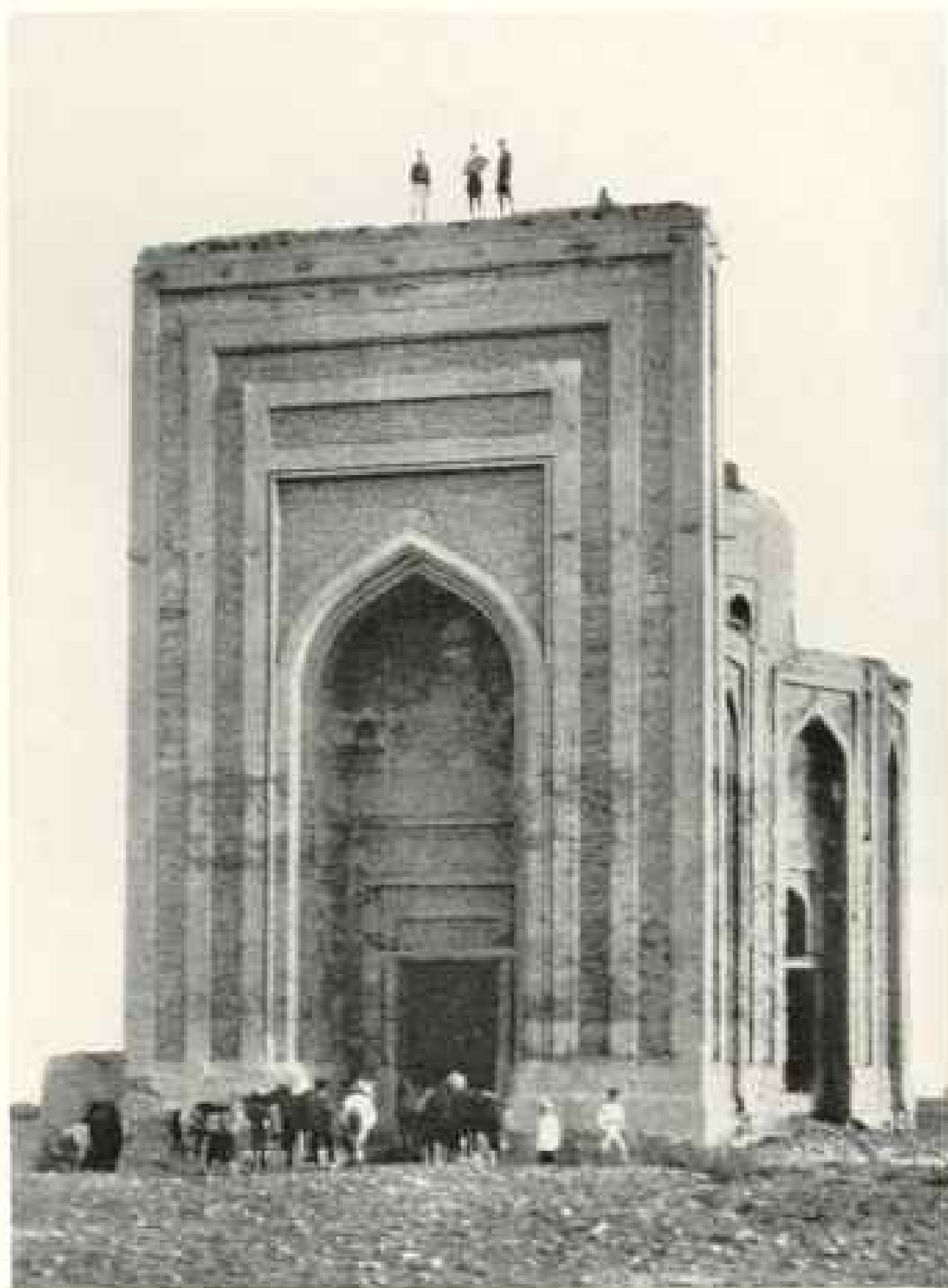
THE PRINCIPAL RUIN AT URGENCH
