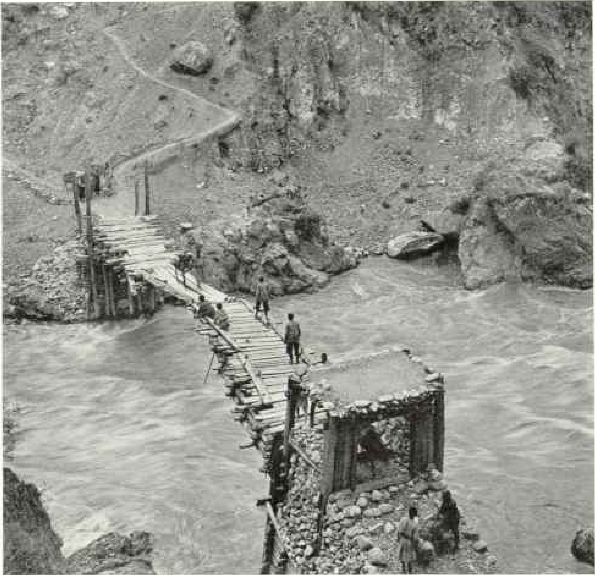
THE CANTILEVER BRIDGE OVER THE SHOU CHU AT SHENDZONG (SEE PAGE 34)
