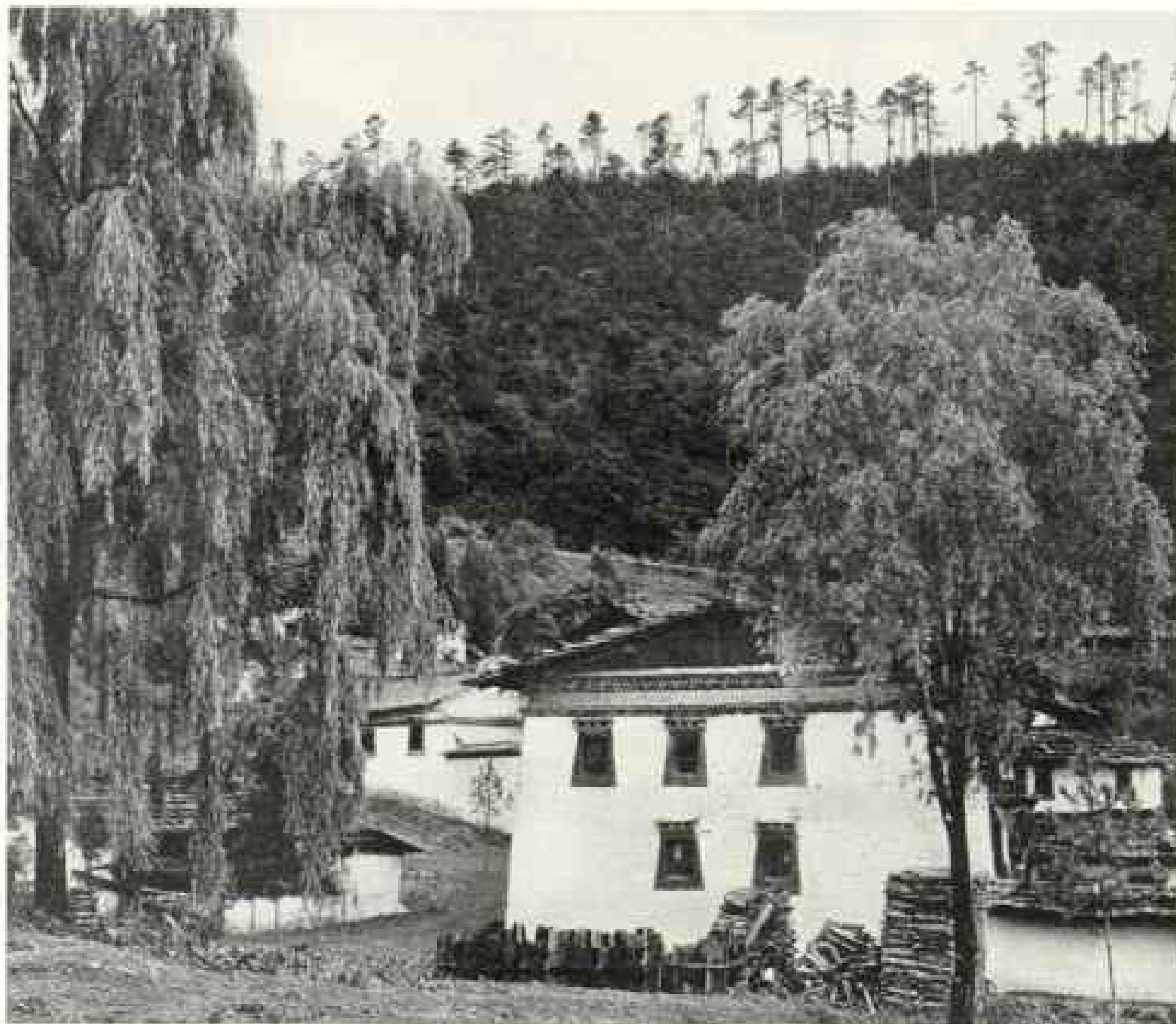
THE OLD CHANTING HALL AT KOPATI MONASTERY, IN MULI TERRITORY
