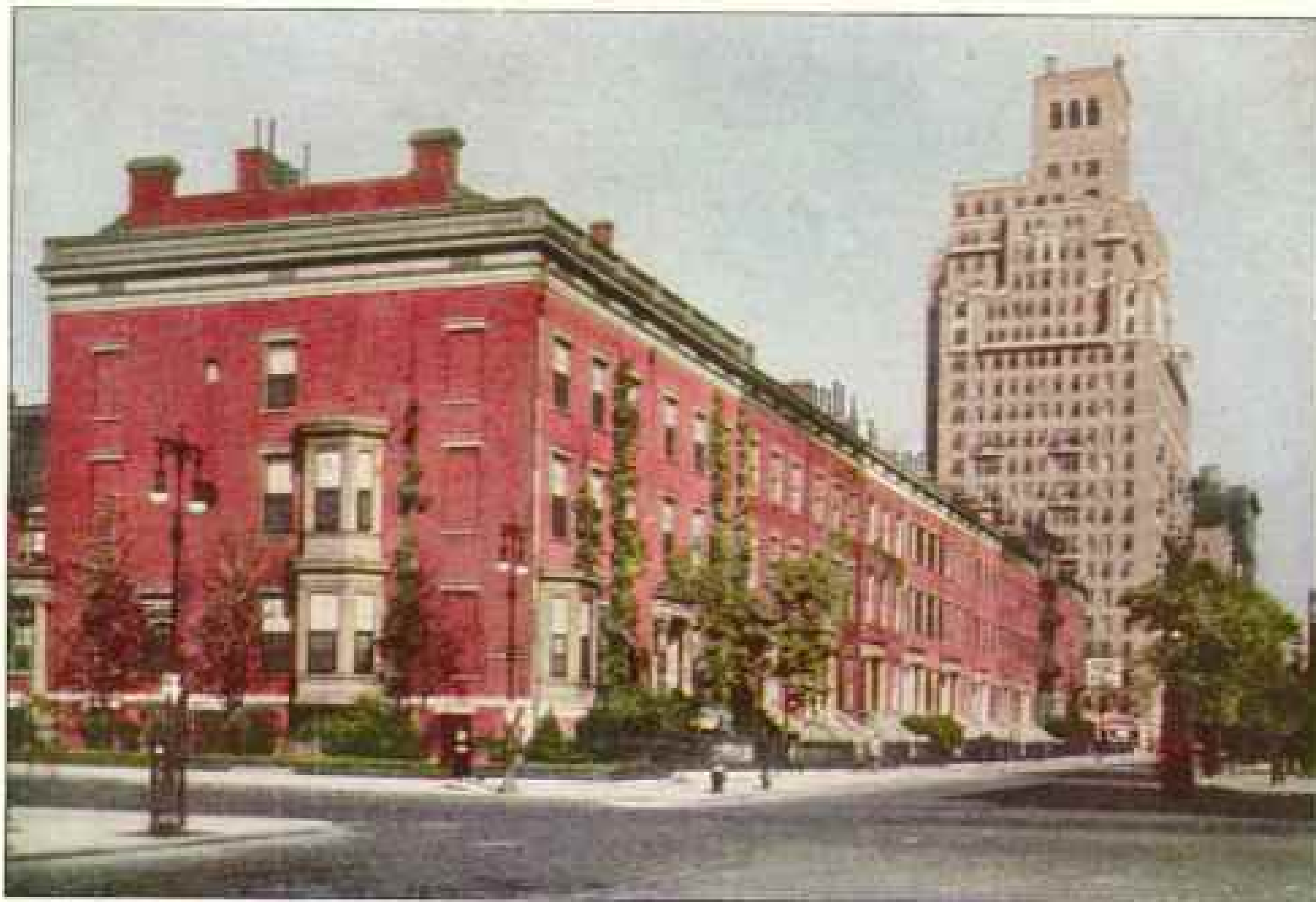
THE OLD AND THE NEW ALONG WASHINGTON SQUARE
