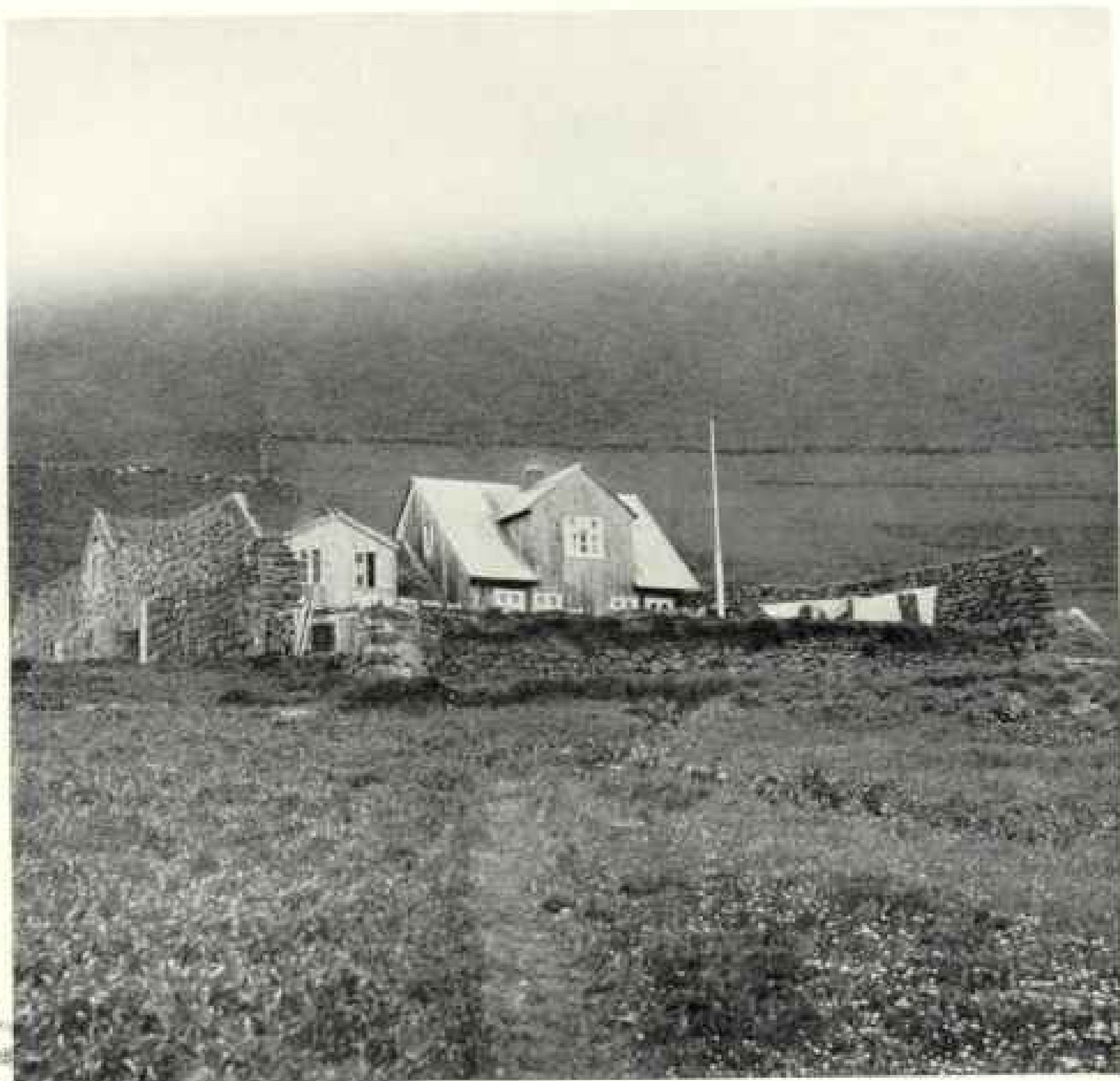
BRACED STONE WALLS DEFLECT THE VIOLENT WINDS
