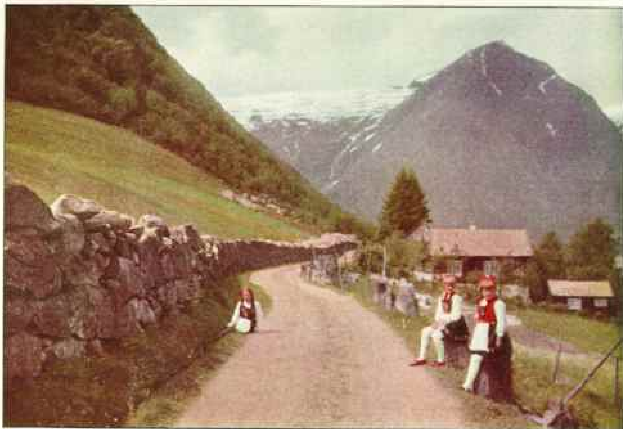
NORWEGIAN ROAD-BUILDING DEMANDS ENGINEERING SKILL.
