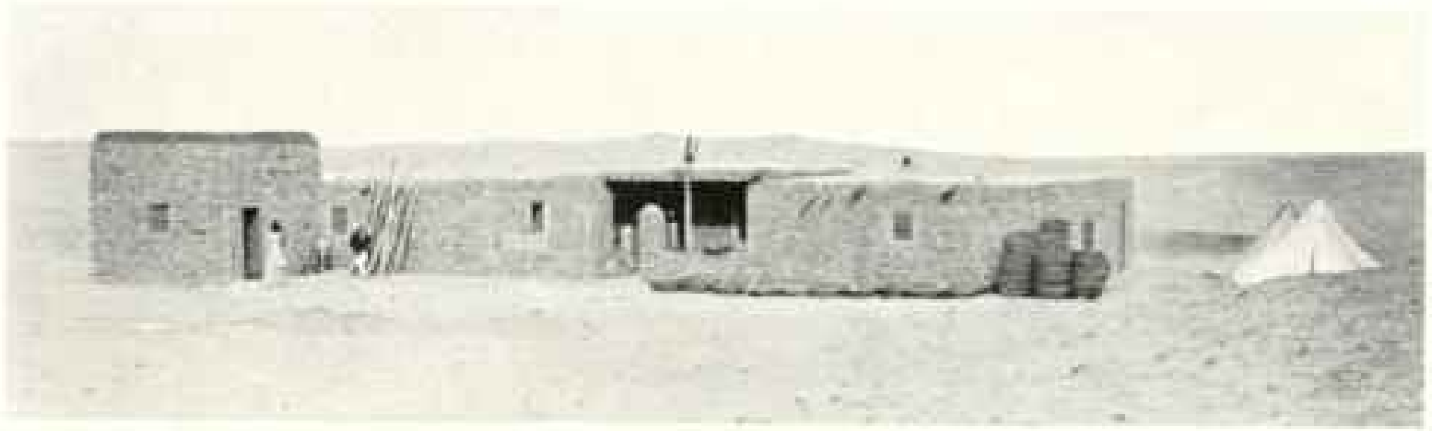
THE EXPEDITION'S HOUSE AT UR IS CONSTRUCTED OF BURNT BRICKS
