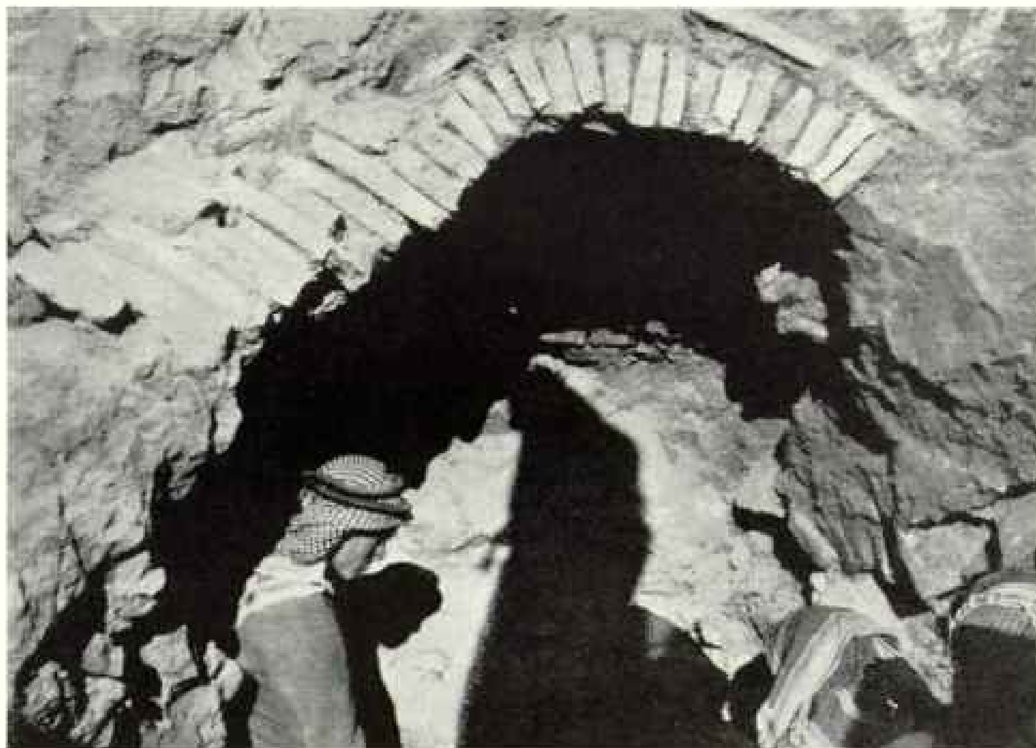
A VAULT OF BRICK DISTINGUISHES THIS ROYAL TOMB AT UR, WHICH DATES FROM THE FOURTH MILLENNIUM B. C.
