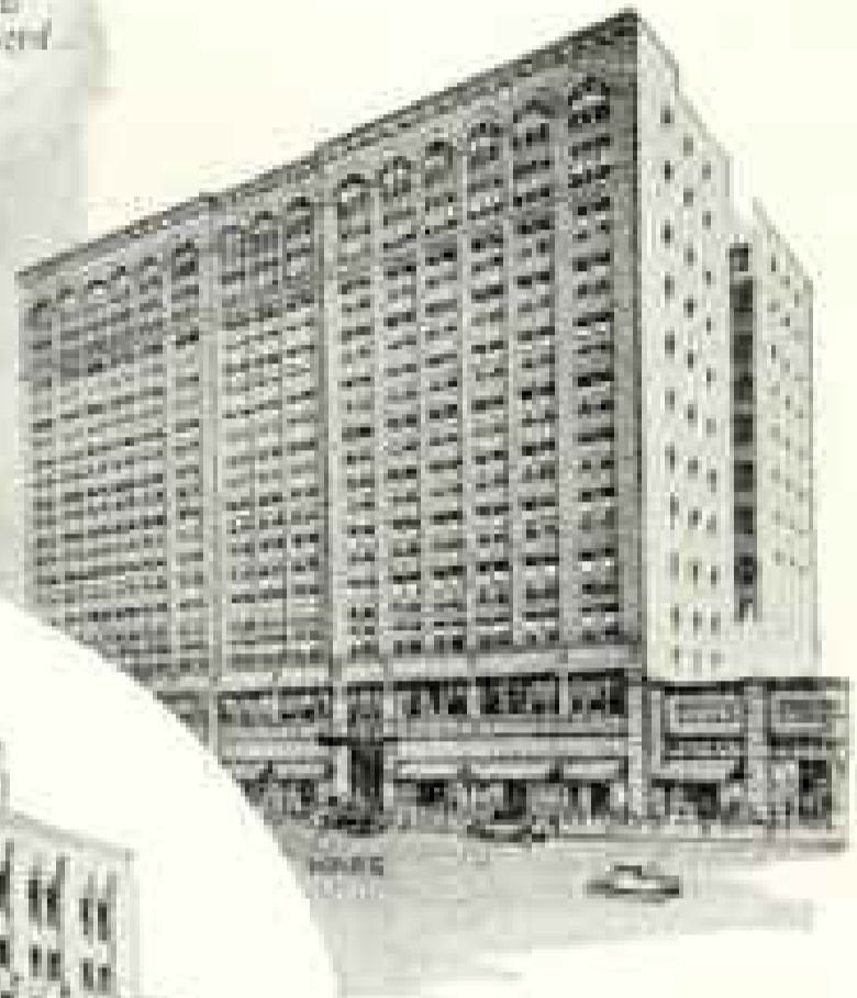
Western Pacific Building Los Angeles, Calif. Owner—L. A. Investment Bldg. Co., Los Angeles Architects—Walker and Tison, Los Angeles Contractors—Los Angeles Investment Co., Los Angeles Business Dealers—Russell- Montgomery Hardware Com- pany, Los Angeles
