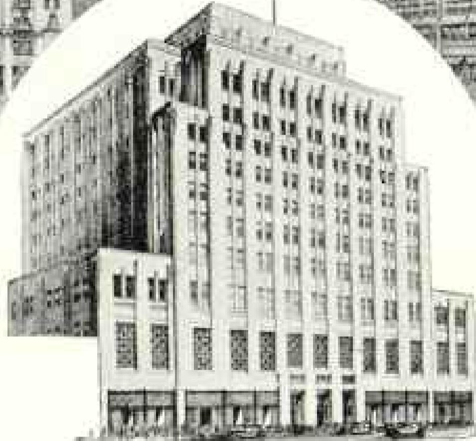
Title Insurance Building Los Angeles, Calif. Architects—John Parkinson & Donald B. Parkinson, Los Angeles Contractors—Sethill Eng. Company, Los Angeles Business Dealers—Russell-Montgomery Hardware Co., Los Angeles
