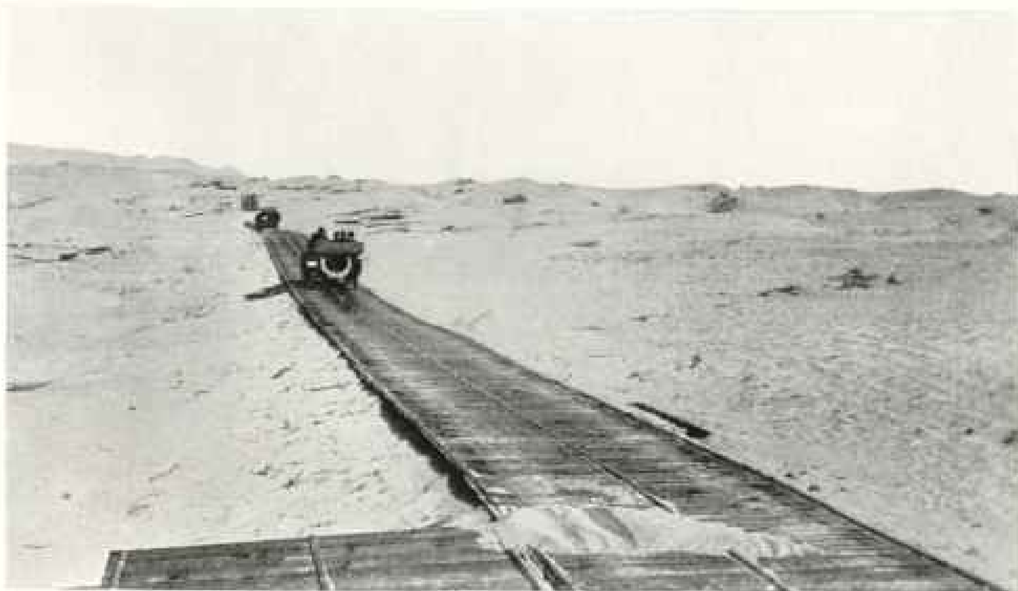
A COMPLETED STRETCH OF PLANK ROAD OVER THE CALIFORNIA DESERT
