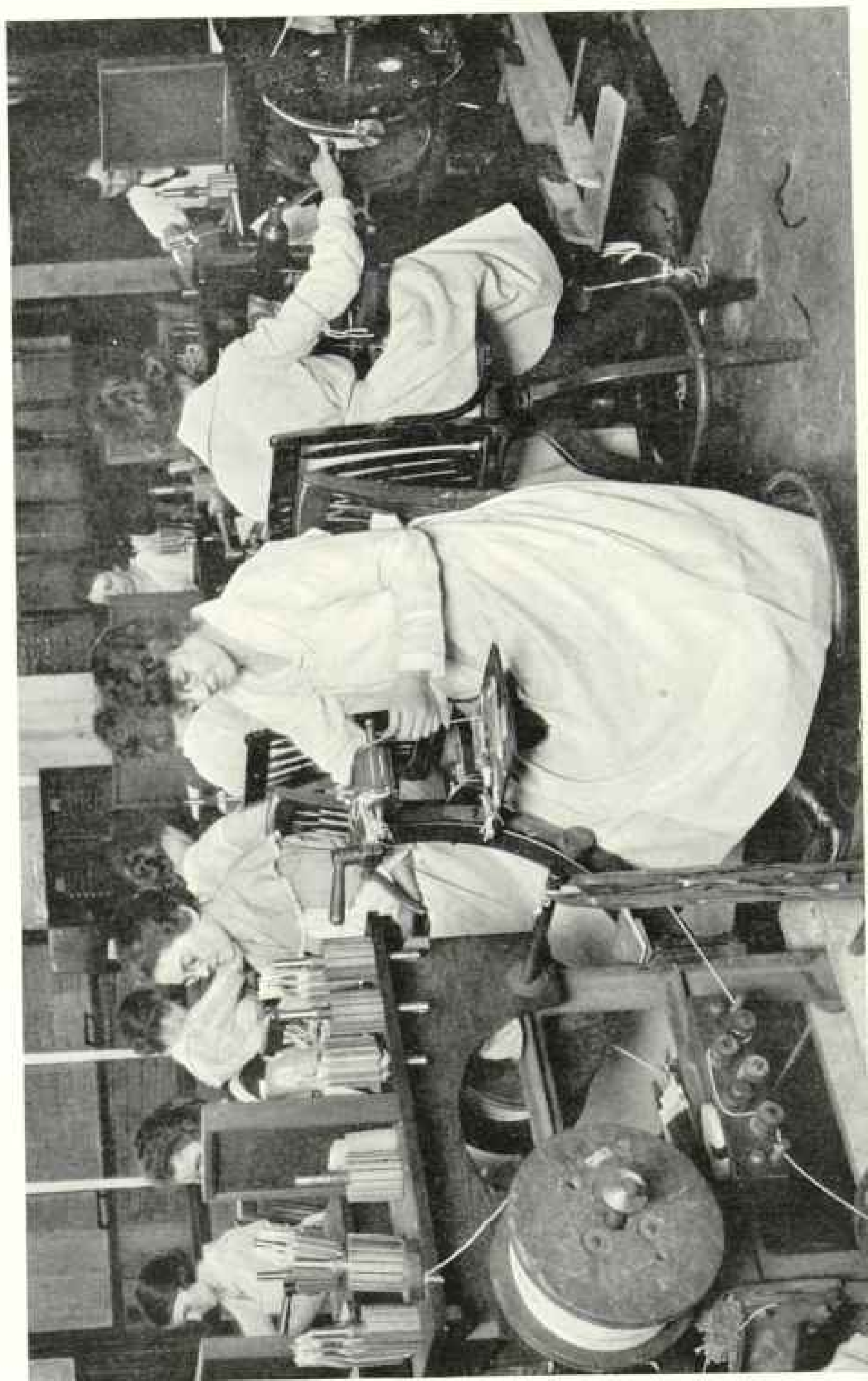
WINDING ARMATURES FOR MOTOR-CAR GENERATORS
