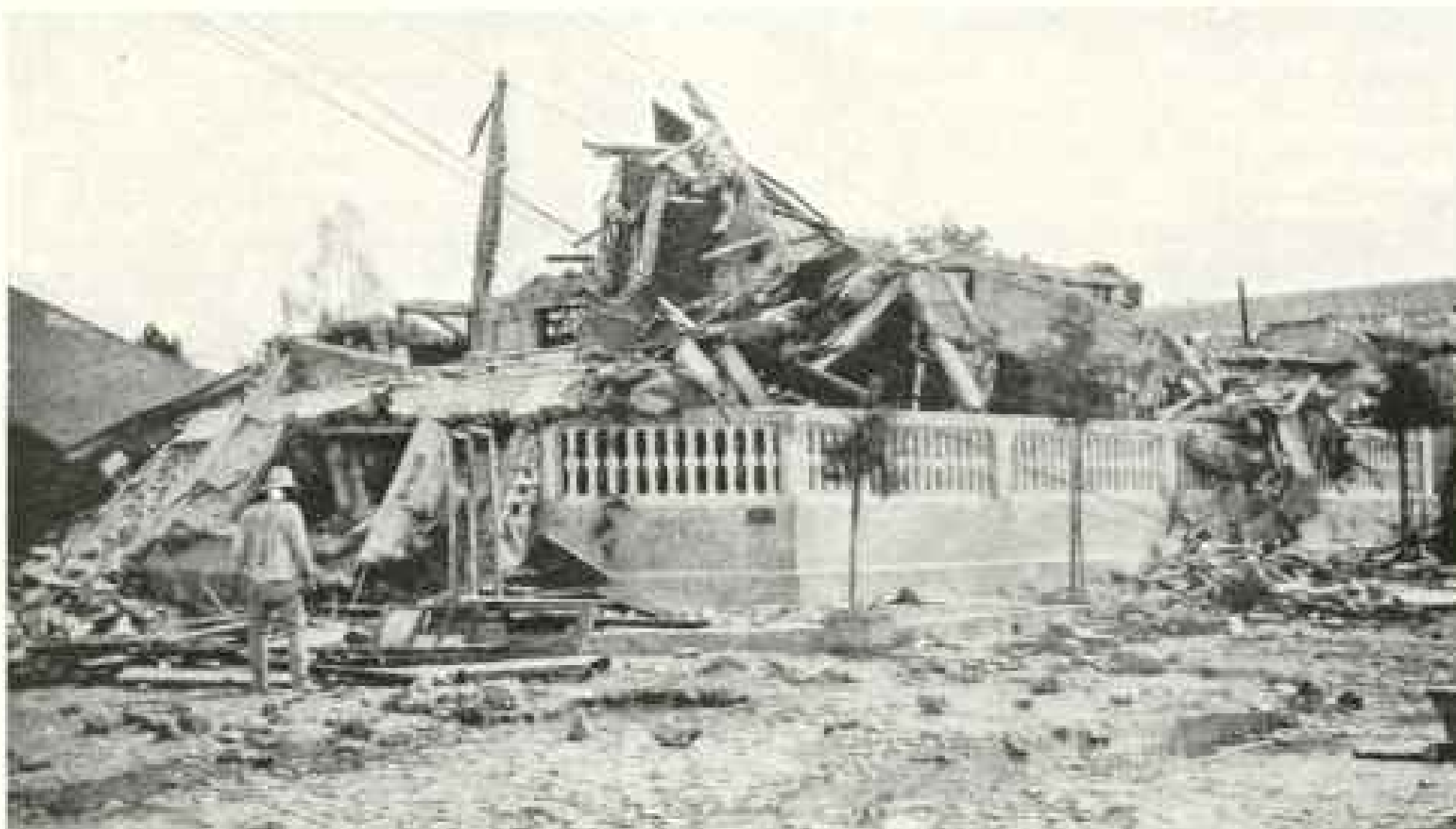
A HOUSE OF LIGHT CONCRETE CONSTRUCTION REDUCED TO A PILE OF DEBRIS BY THE EARTHQUAKE: SAN SALVADOR
