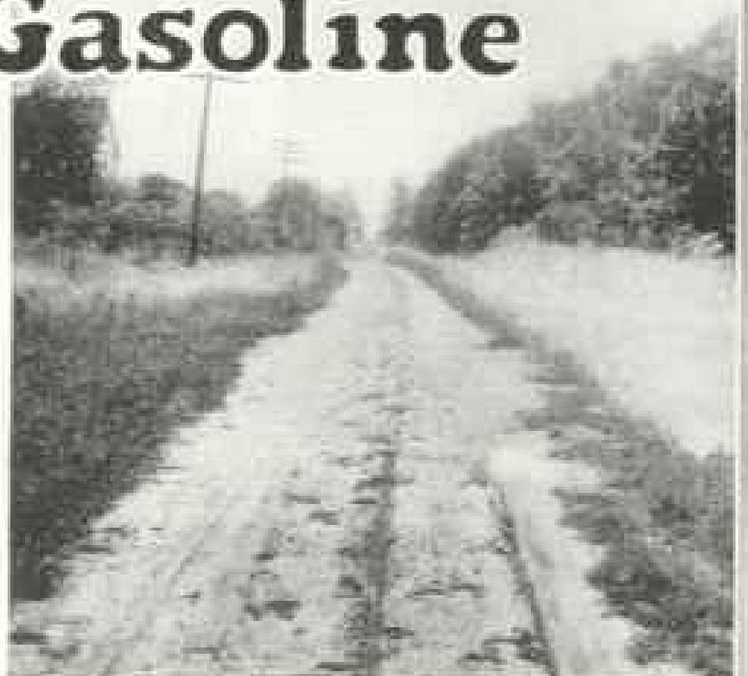
5.78 miles per gallon of gasoline on this earth road—less than half the mileage obtained on the concrete road opposite.
