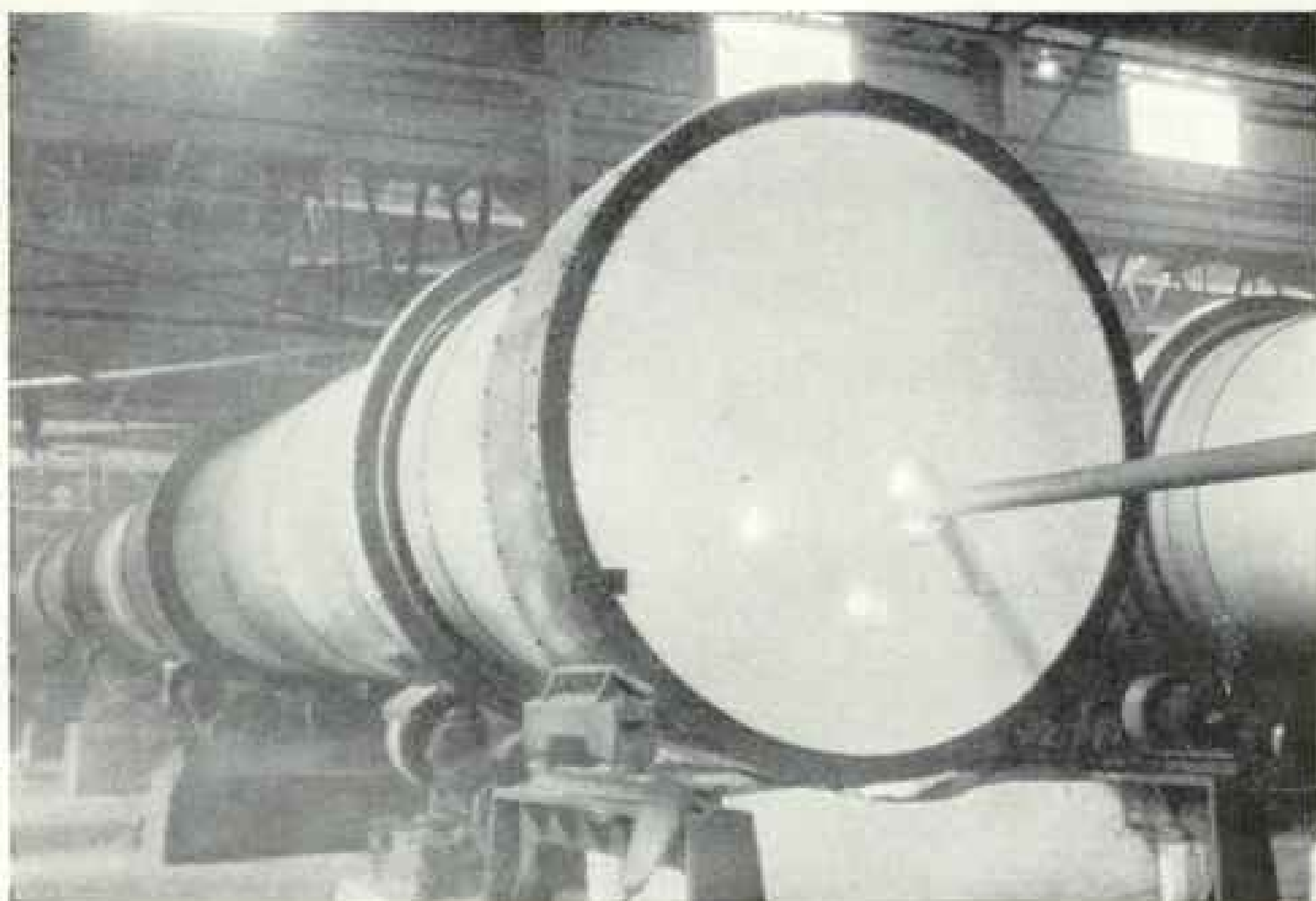
A ROTARY CEMENT KILN.
