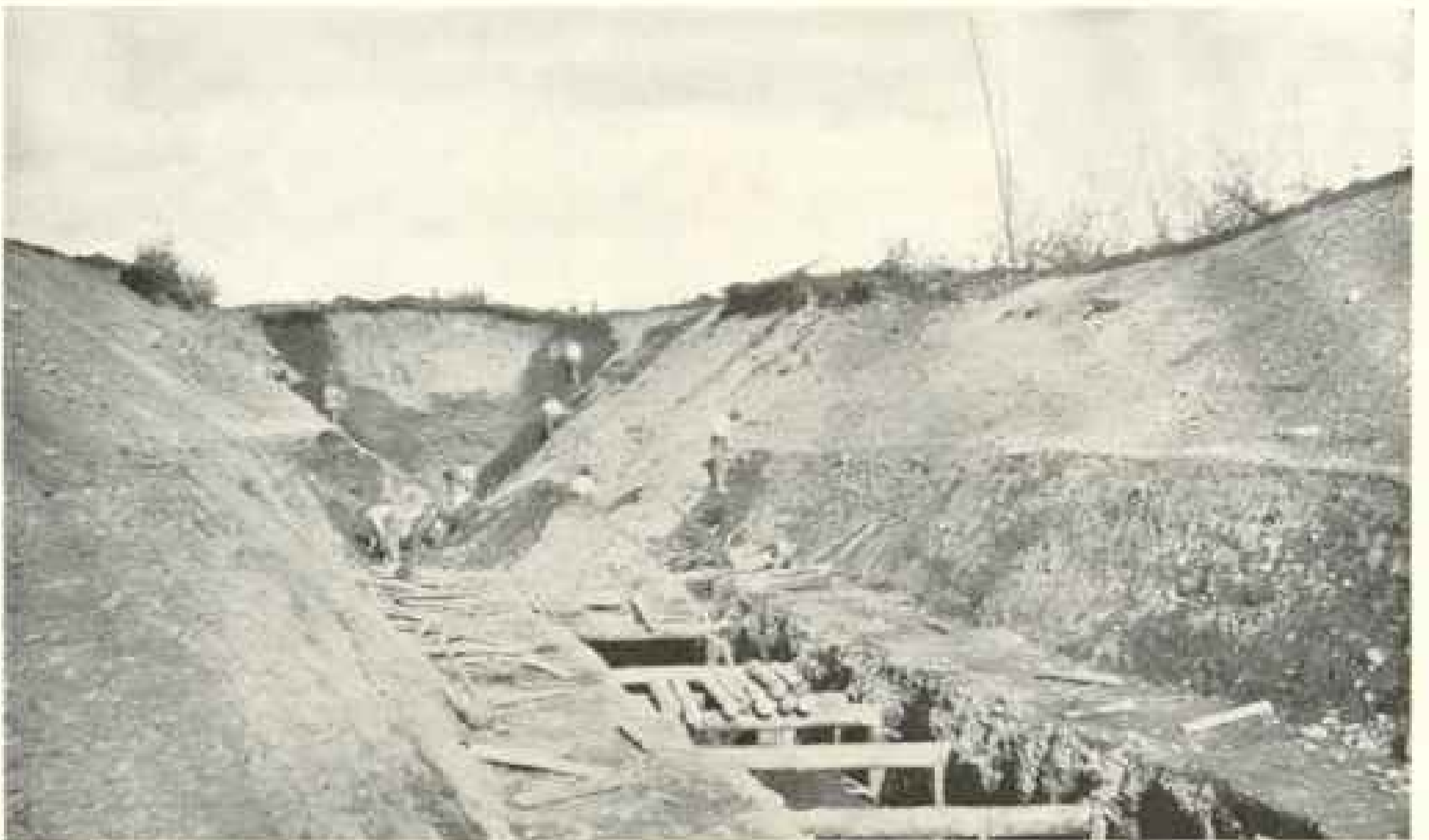
METHOD OF TRAPPING CUTS INTO SMALL CARS
