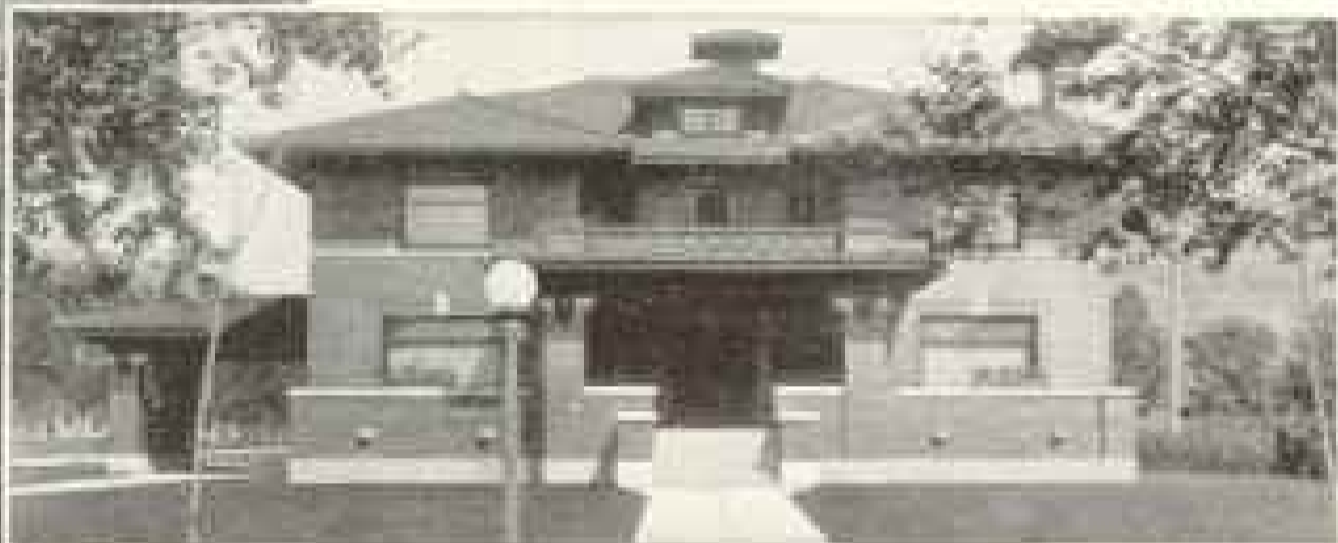
RESIDENCE OF J. H. KEITH, MISSOULA, MONT. Hy-tex No. 550 Brick Lans & Hains, Helena, Mont. Architects
