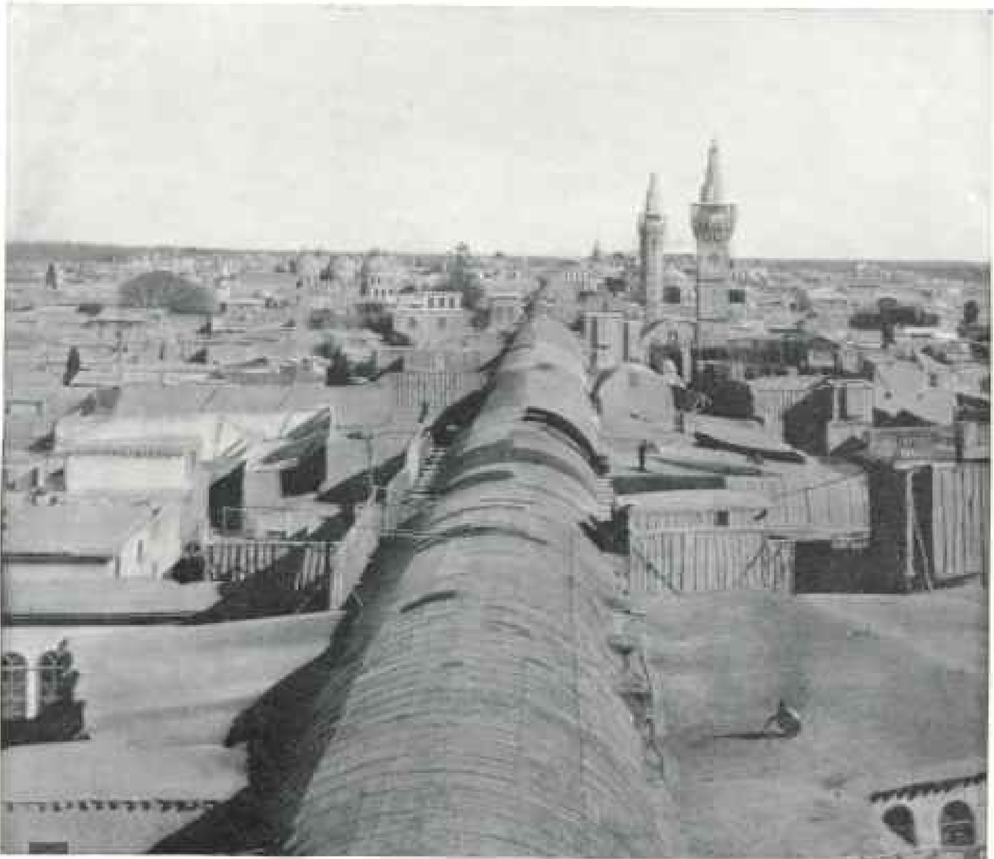
ROOF OF "STRAIGHT" STREET IN DAMASCUS
