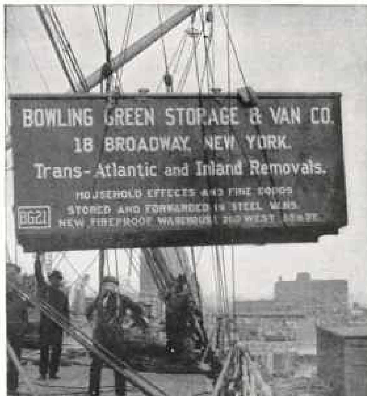
HOISTING LIFT-VAN ON BOARD STEAMSHIP
