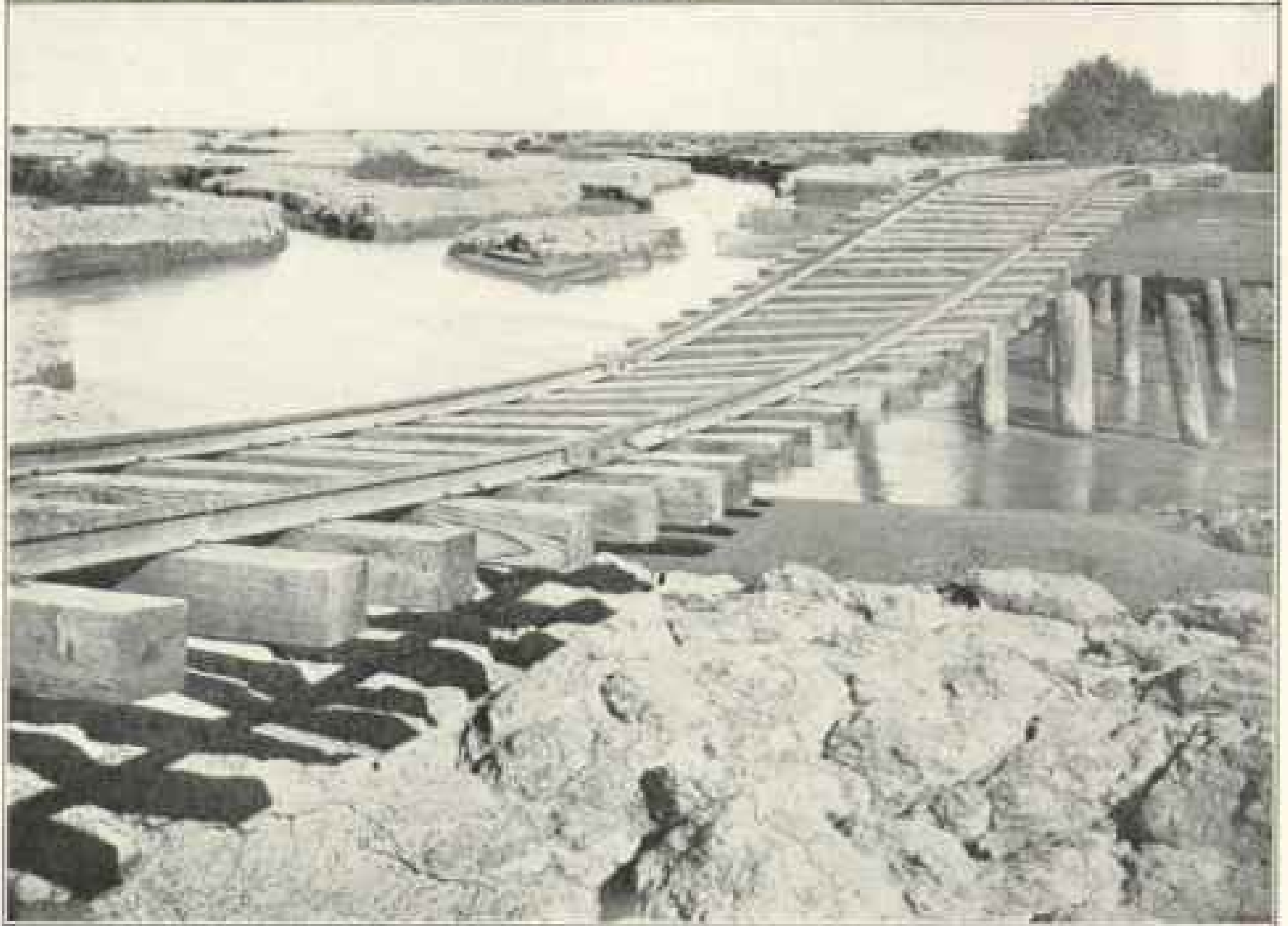
A Section of the Imperial Valley Which Was at First Inundated and Then Left High and Dry by the Deepening Channel
