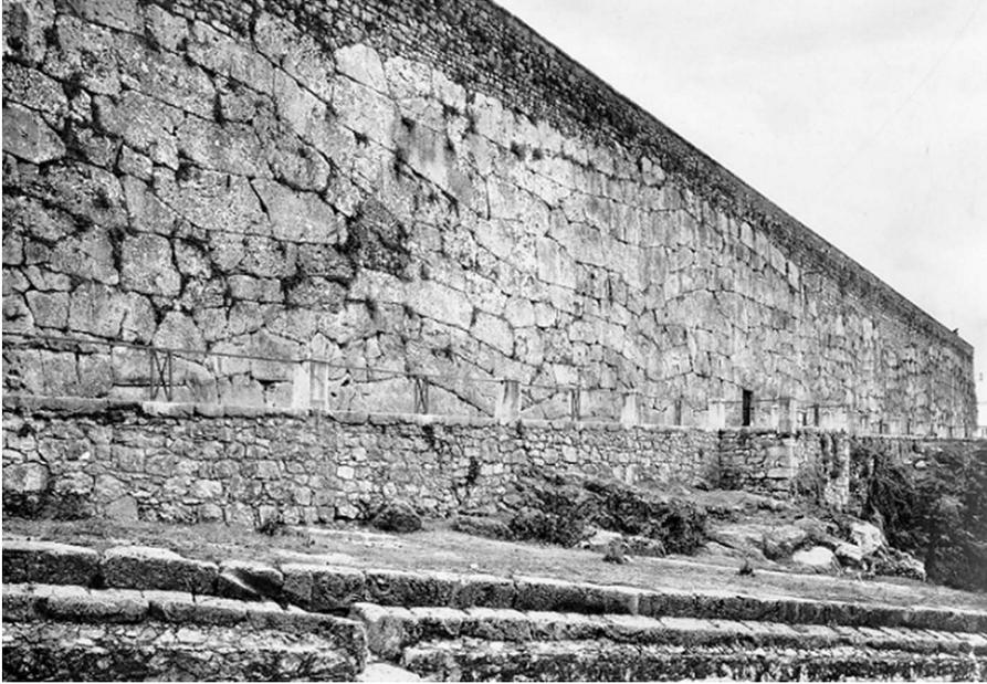
**Figure 10.6:** Polygonal walls of the Alatri Acropolis, Italy.
