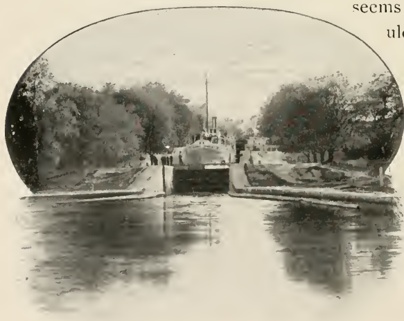
READY TO STEP DOWN AND OUT.
