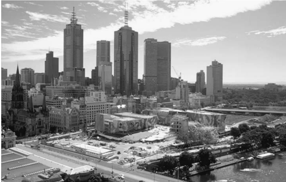
FIGURE 16.1. Federation Square, Melbourne, civic complex during construction, 5 March 2001.
