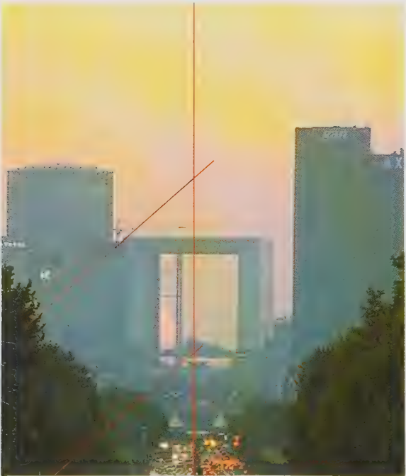
16. View of the Grande Arche looking west. The 6 degrees deviation of the Grande Arche's axis from that of the Historical Axis is obvious. This produces an orientation of 32 degrees north-of-west towards the sunset horizon, matching the sunset on 24 June (see plate 15).
