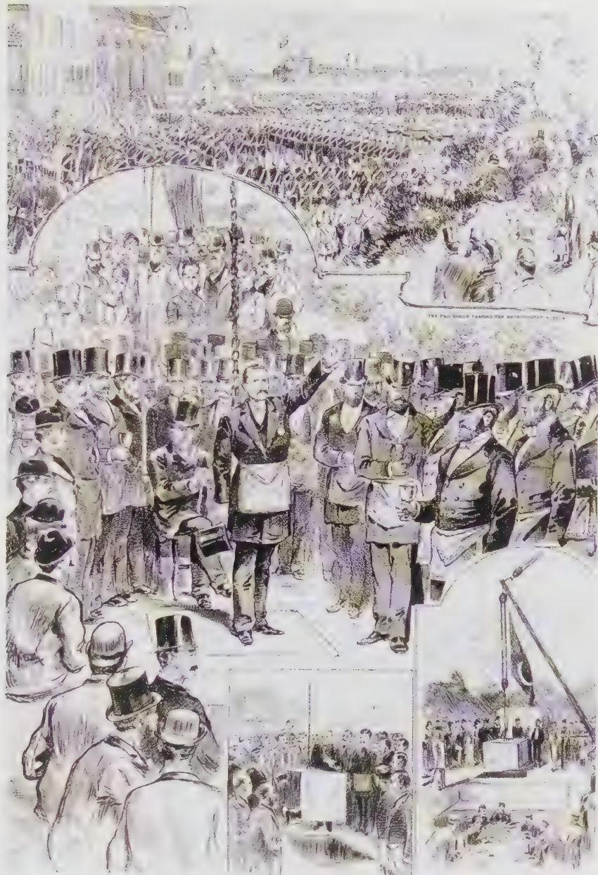
41. The Masonic foundation-laying ceremony for the New York obelisk in 1880 during which the Grand Master linked Freemasonry to ancient Egypt.
