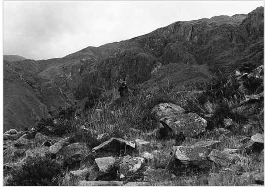
Damage at Sacsayhuaman.
